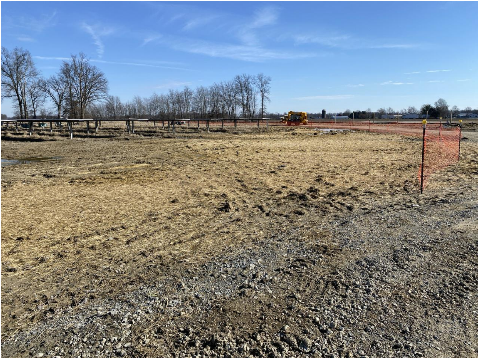
Photo 2: Access road shoulder protection, Straw mulch stabilization
