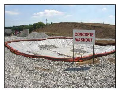
Concrete washout areas are designated locations within a construction site that are either a prefabricated unit or a designed measure that is constructed to contain concrete washout. Concrete washout systems are typically used to contain washout water when chutes and hoppers are rinsed following delivery.
