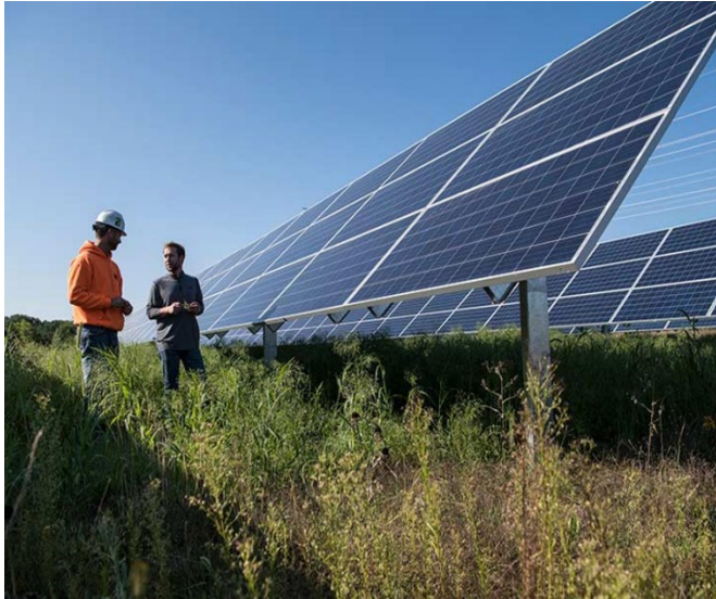
Low-impact solar project installation of the Aurora Solar Project with native plant growth under the solar panel area. Photo from the National Renewable Energy Laboratory.
