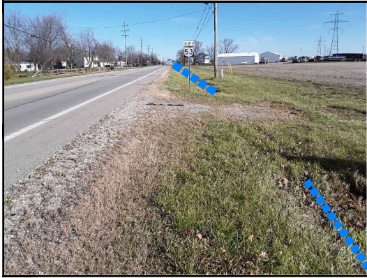
TYPE 2: EXISTING GRAVEL ACCESS LOCATION WITH 12" CMP CULVERT WITHIN THE ROW OF W FREMONT ROAD (SR-53). INSTALL ADDITIONAL GRAVEL TO FACILITATE CONSTRUCTION ACCESS.
