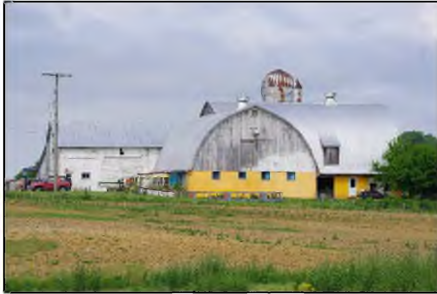
Photograph 5-15: Overview of original wood-framed barn with Gothic-arch barn additions (45b) and silo (45c) rear
