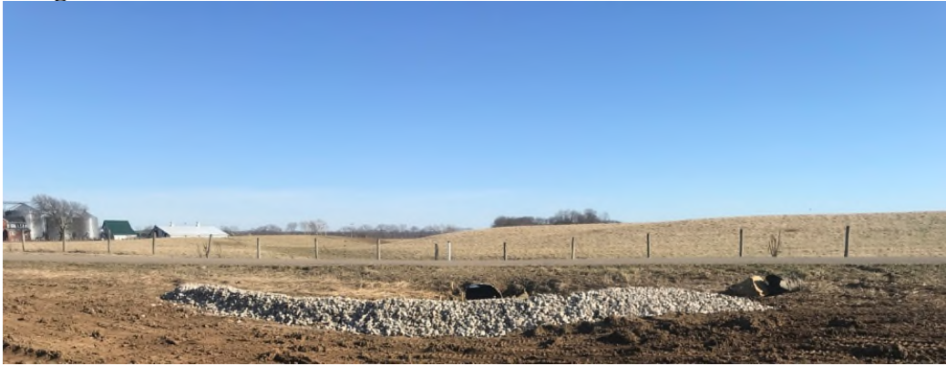
Image 1: Rock Ditch Check Feature at the Yellowbud Site
