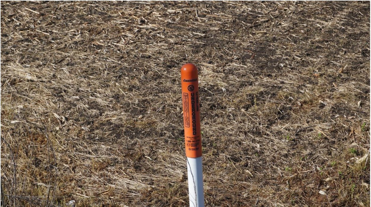
Fiber optic cable marker in SW Quad at toe of railroad embankment (Not shown, similar marker in SE quadrant)
