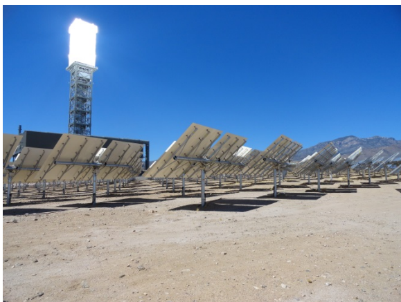
Figure 6. Reflectors in inner circle of PT.
