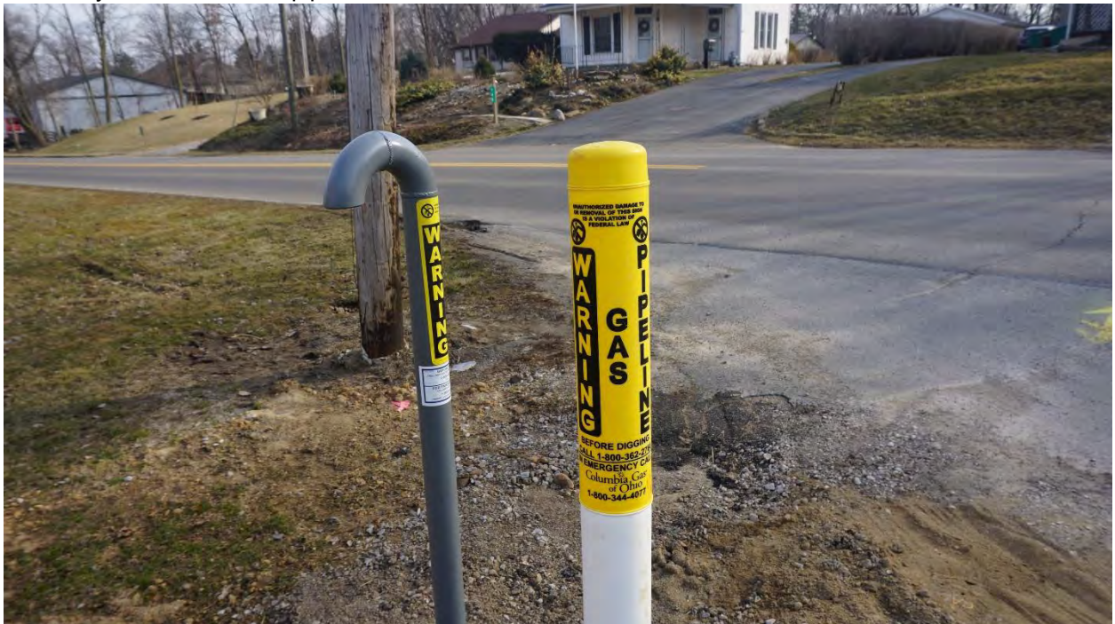
Gas utility marker and vent pipe in NE Quad
