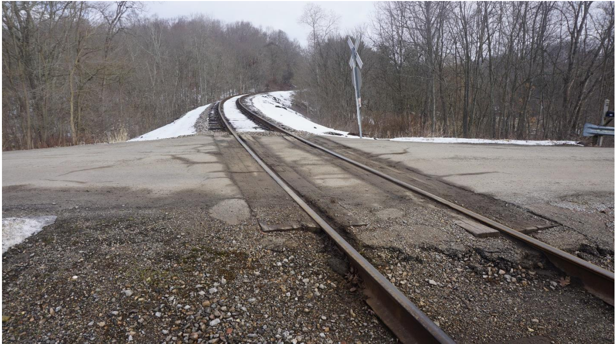
SW Quad viewing north (4 gauge rods in curve to be removed and 16 ties installed)
