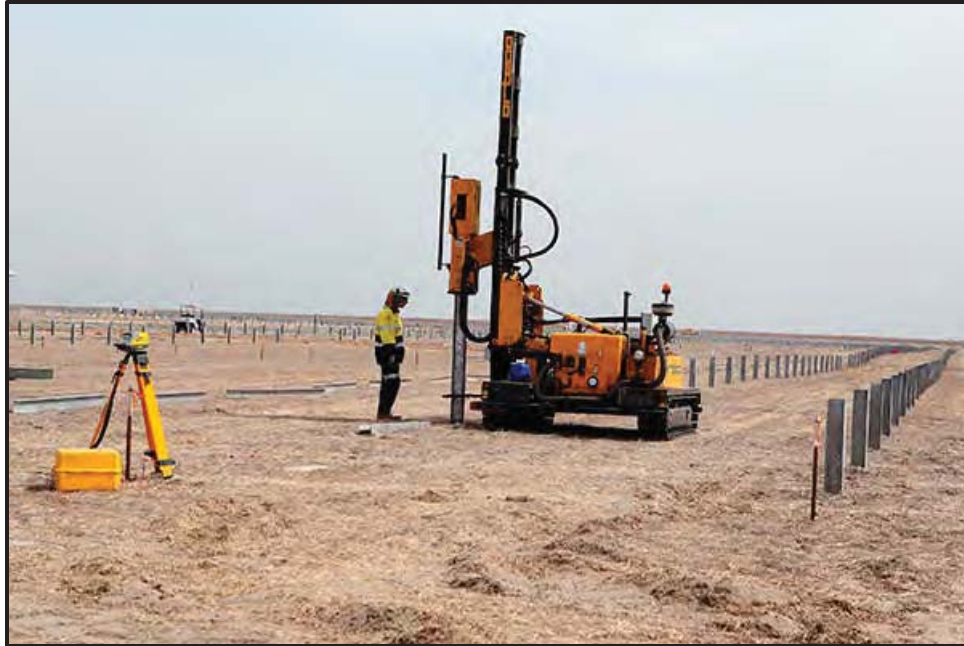
Figure 3. Example of racking being driven into the ground by a pile driver during construction. 1
