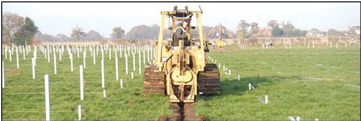
Figure 4. Example of trenching associated with the electrical collection system. 2
