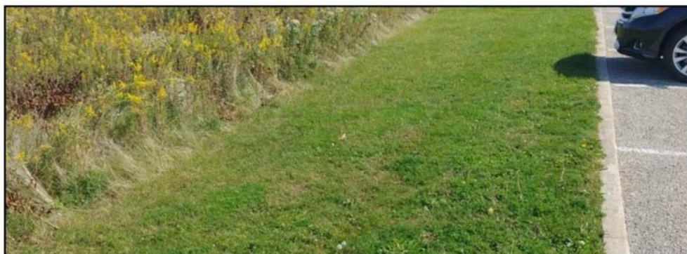
Figure 2.2.4 Depiction of Impervious Surface Disconnection to Establish Sheet Flow to a Conservation Area
