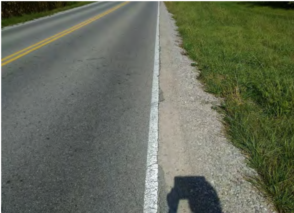
PHOTO 12: Pavement distress (edge failure) on Watkins Road, looking north.
