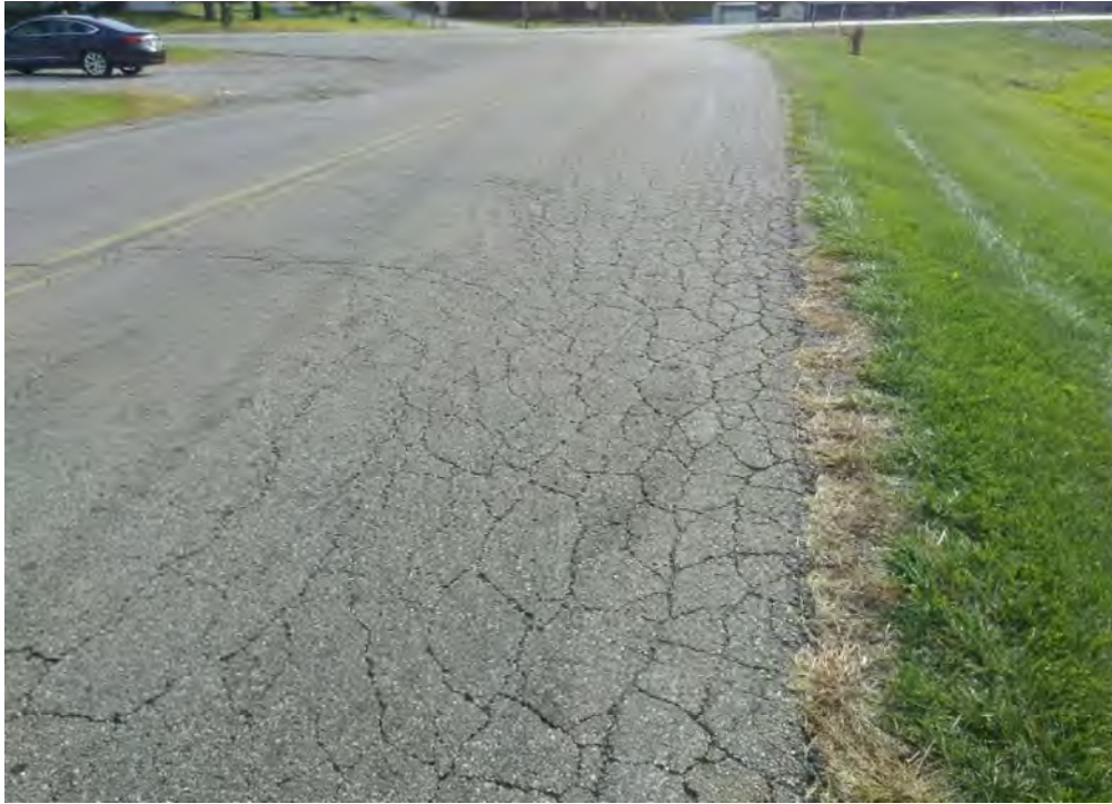
PHOTO 35: Pavement distress (alligator cracking) on York Road, looking south.
