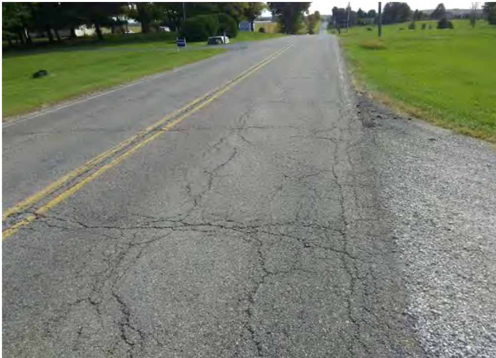
PHOTO 22: Pavement distress (transverse and longitudinal cracking) on York Road, looking south.
