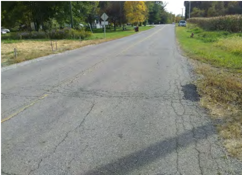
PHOTO 32: Pavement distress (transverse, longitudinal and alligator cracking) on York Road, looking south.
