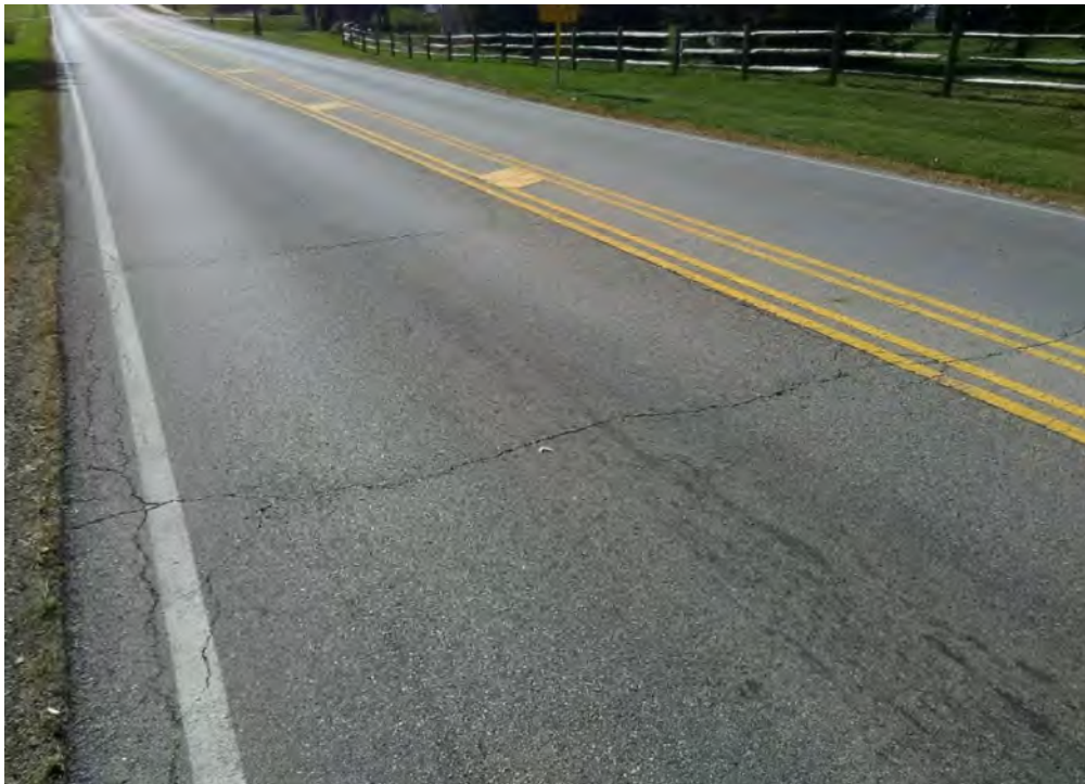
PHOTO 4: Pavement distress (transverse cracking) on Watkins Road, looking south.
