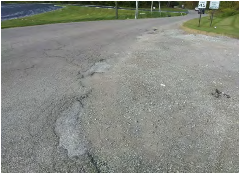
PHOTO 34: Pavement distress (edge failure) on York Road, looking north.
