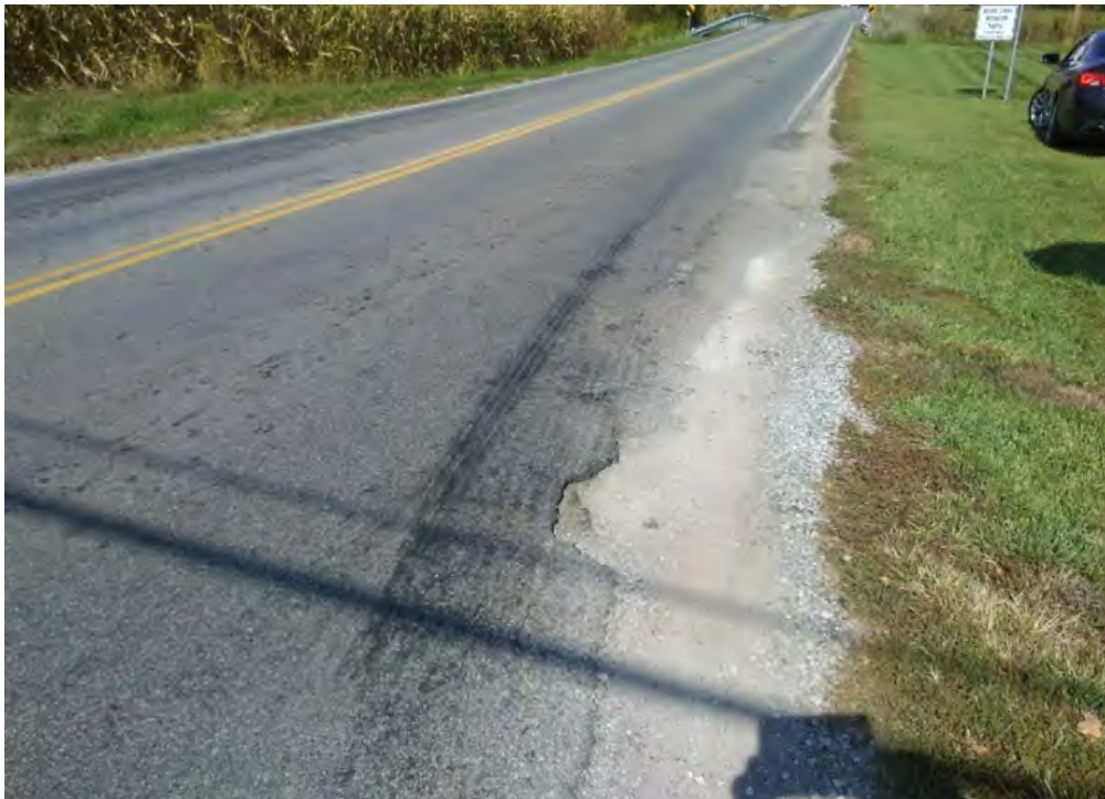
PHOTO 6: Pavement distress (edge failure) on Watkins Road, looking north.
