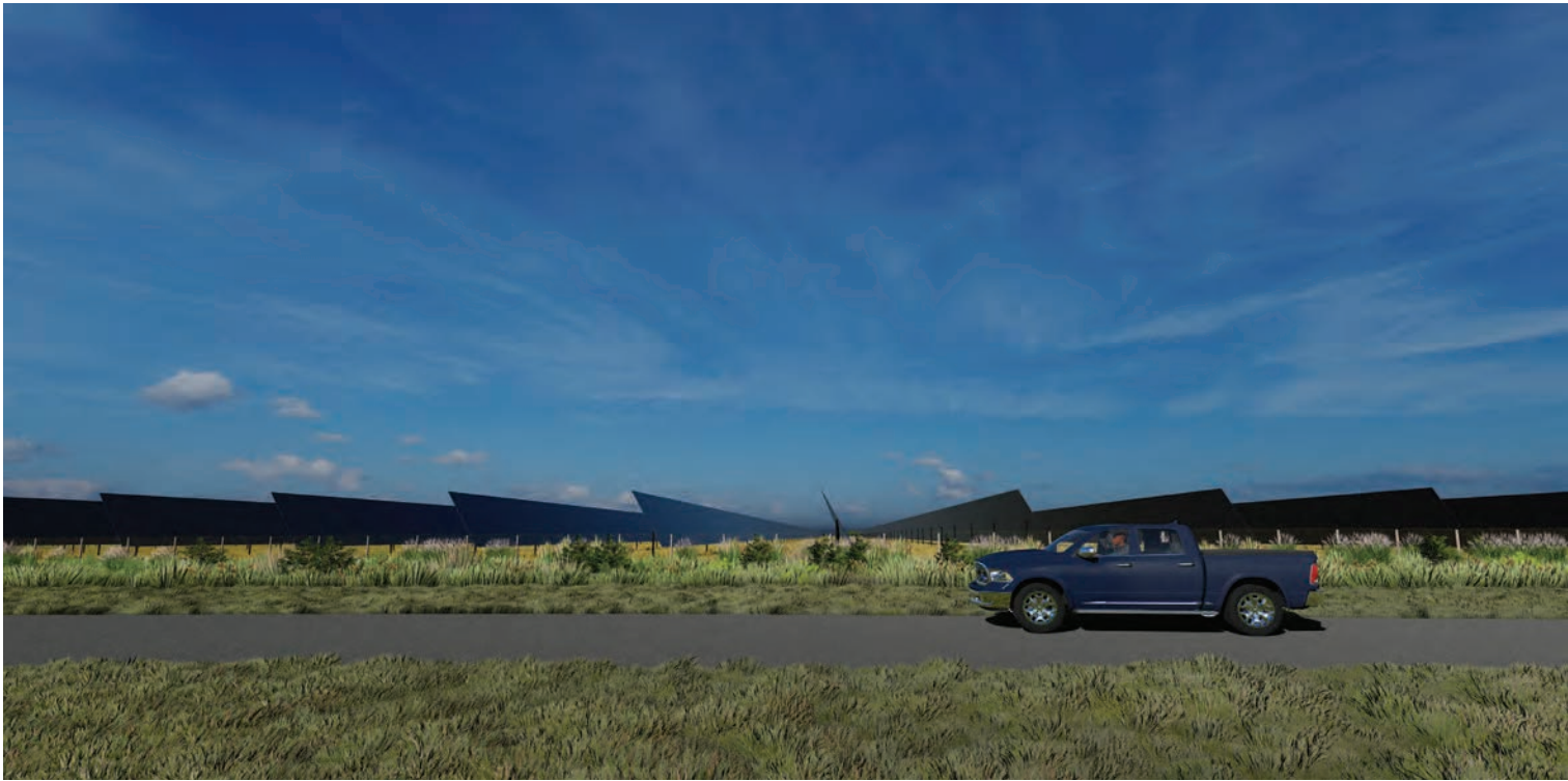
LOW DENSITY PLANTING - POLLINATOR MIX SOLAR PANELS FROM A 30' DISTANCE ON AN EAST-WEST ROAD. PANELS SHOWN AT MAXIMUM 15' HEIGHT, 60 DEGREE TILT.
