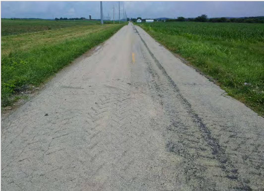
PHOTO 9: Pavement distress (cracked pavement) over culvert on Lower Twin Road, looking east.
