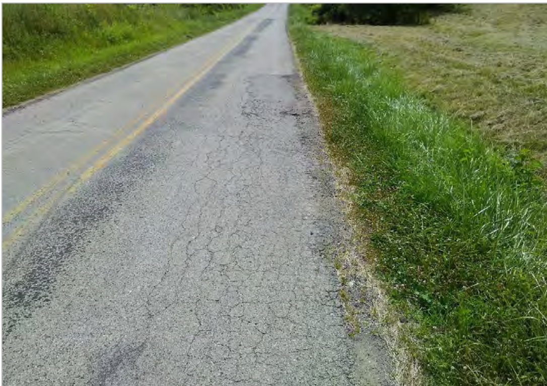
PHOTO 2: Pavement distress (edge deterioration) on Lower Twin Road, looking east.
