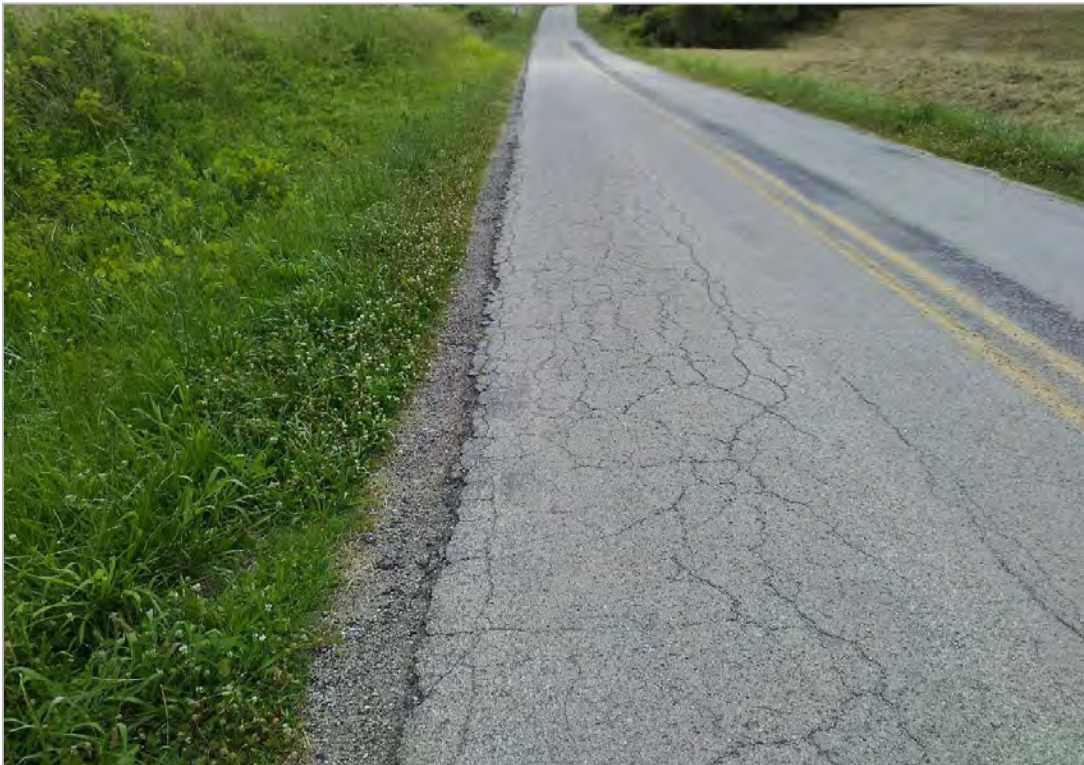
PHOTO 3: Pavement distress (edge deterioration) on Lower Twin Road, looking east.
