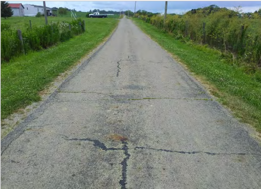
PHOTO 24: Pavement distress (cracked pavement) over culvert on Rolfe Road, looking west.
