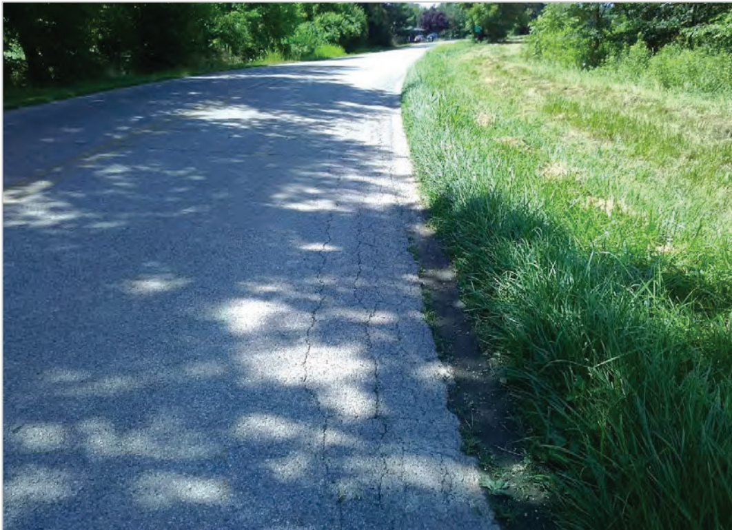
PHOTO 39: Pavement distress (edge deterioration) on Rapid Forge Road, looking north.
