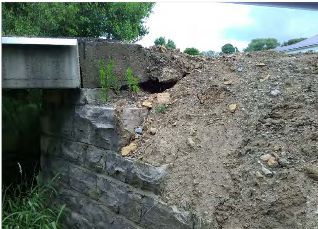
PHOTO 16: View of east bridge (7130570) abutment and embankment erosion on Moxley Road.
