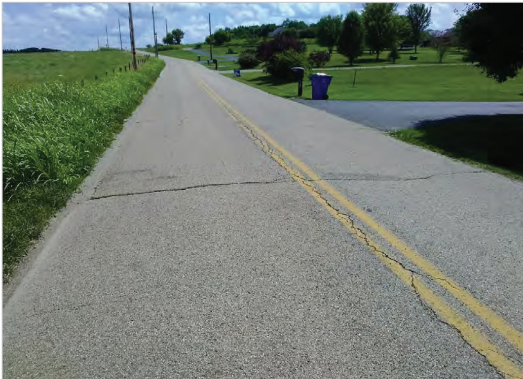
PHOTO 33: Pavement distress (cracked pavement) over culvert on Rapid Forge Road, looking south.
