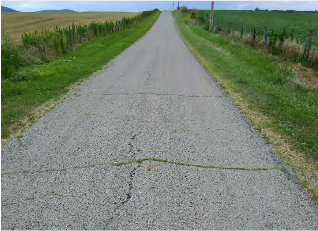
PHOTO 23: Typical pavement distress (transverse cracking) on Rolfe Road, looking south.
