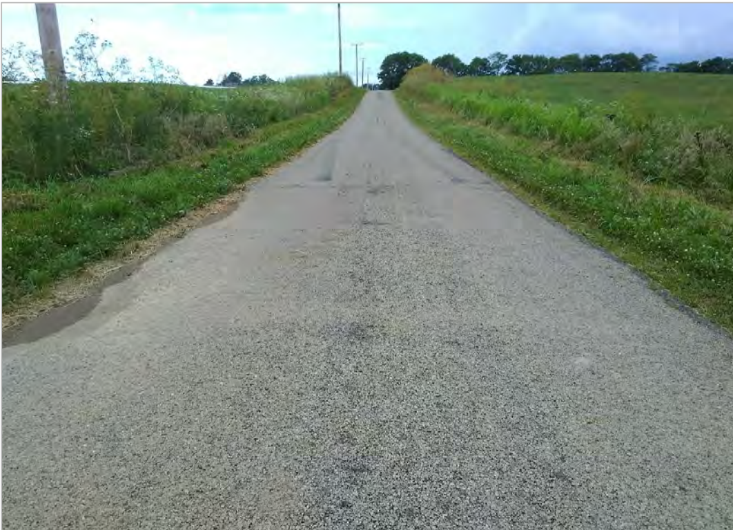
PHOTO 26: Pavement distress (depressed pavement) over culvert on Rolfe Road, looking west.
