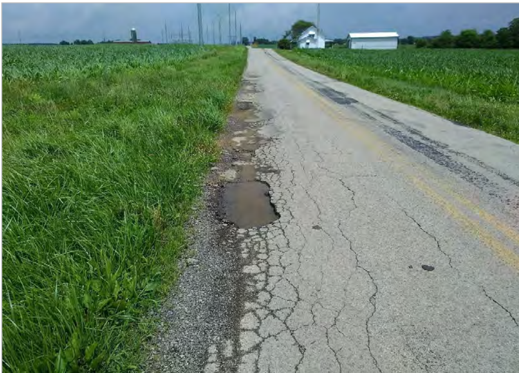
PHOTO 12: Pavement distress (edge failure) on Lower Twin Road, looking east.
