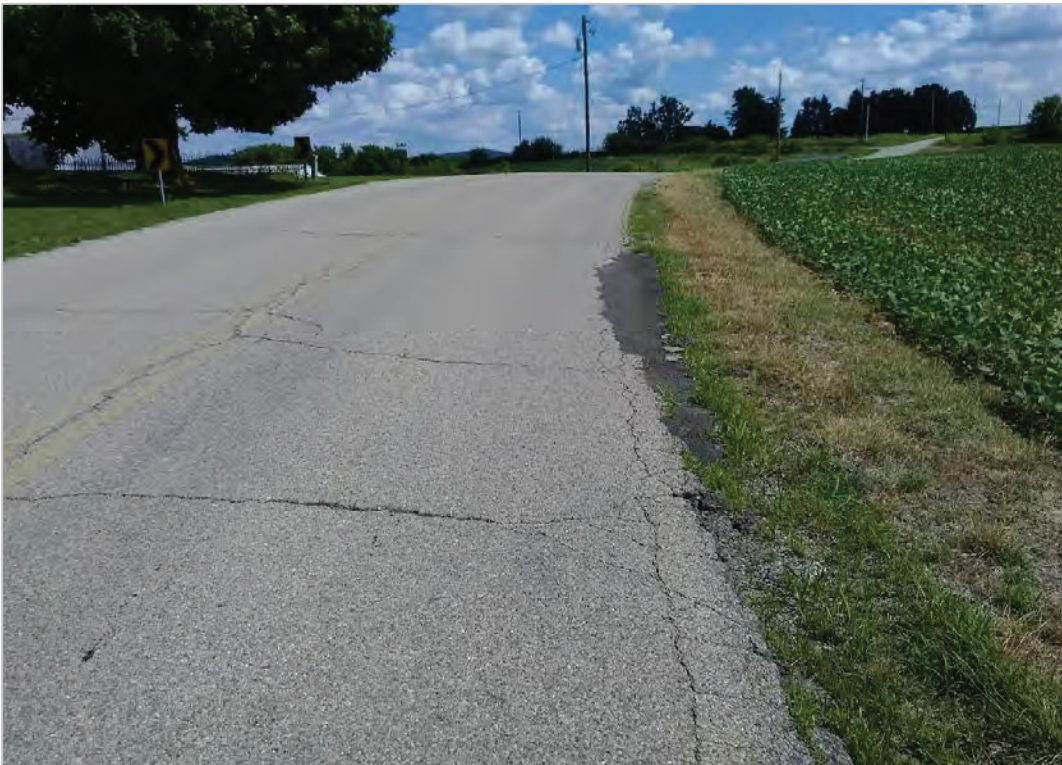
PHOTO 38: Pavement distress (edge failure and repaired pothole) on Rapid Forge Road, looking south.
