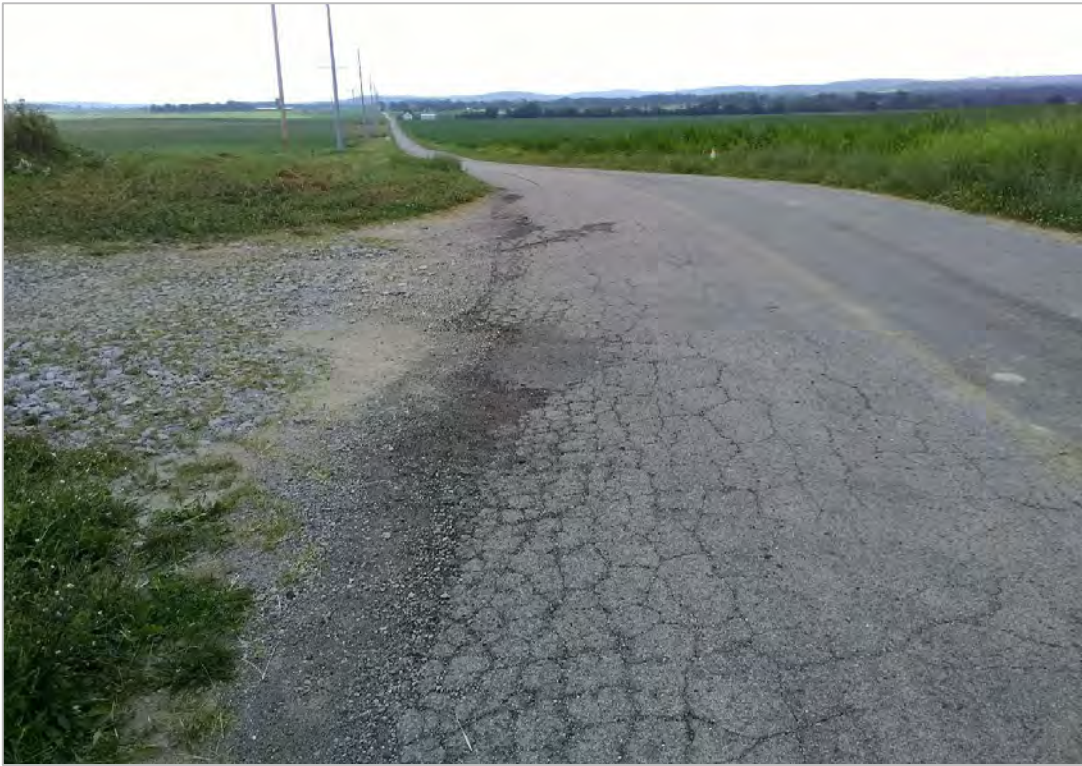
PHOTO 5: Pavement distress (edge deterioration and pothole repair) on Lower Twin Road, looking east.
