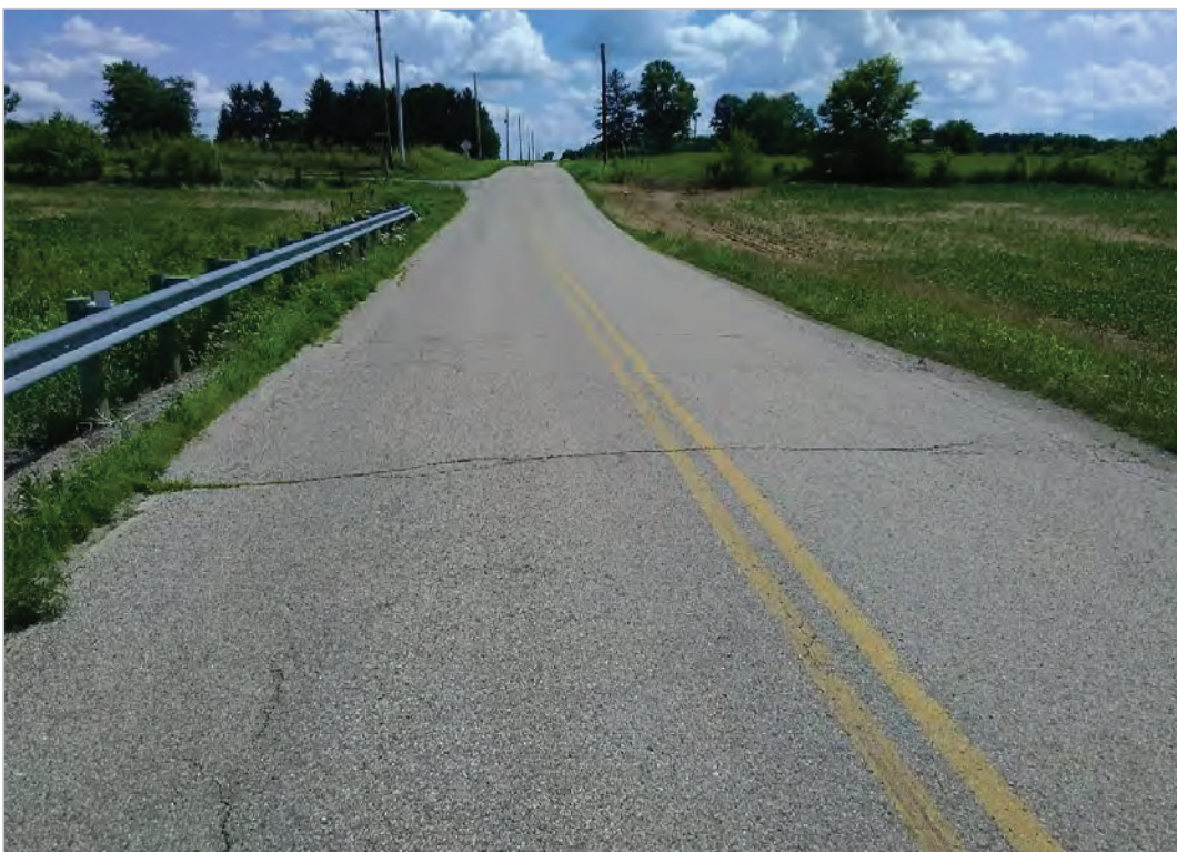
PHOTO 34: Pavement distress (cracked pavement) over culvert on Rapid Forge Road, looking south.
