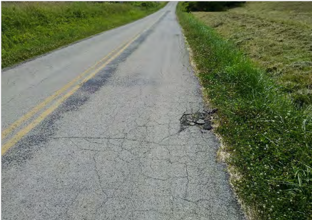
PHOTO 1: Pavement distress (edge failure) on Lower Twin Road, looking east.
