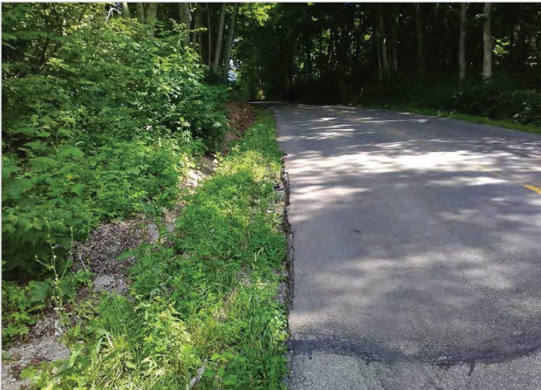
PHOTO 40: Pavement distress (edge failure) and shoulder erosion on Rapid Forge Road, looking south.
