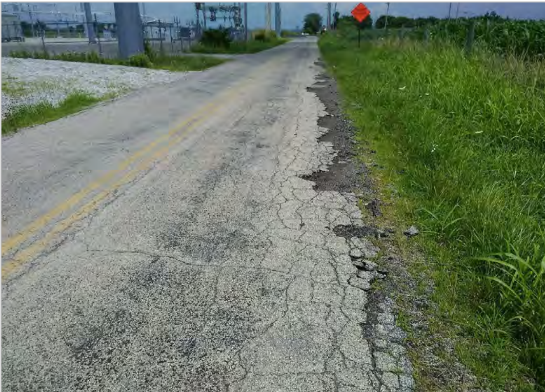
PHOTO 14: Pavement distress (edge failure) on Lower Twin Road, looking east.
