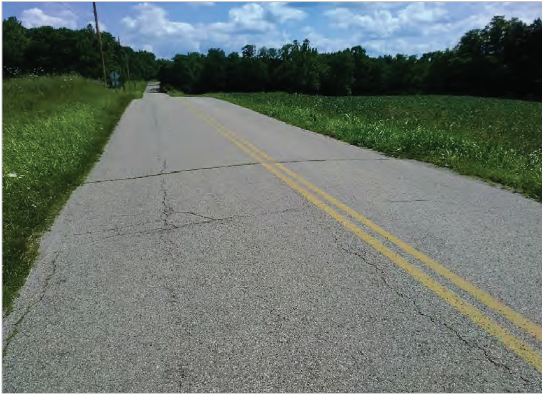
PHOTO 31: Pavement distress (cracked pavement) over culvert on Rapid Forge Road, looking south.
