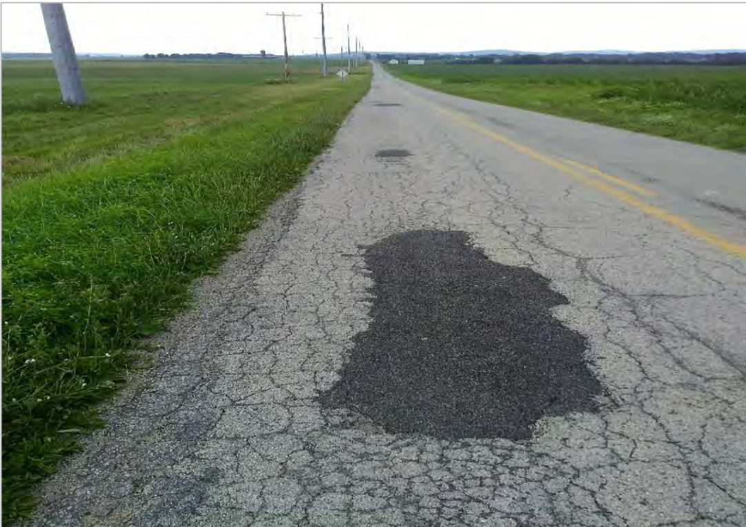
PHOTO 6: Pavement distress (pothole repair) on Lower Twin Road, looking east.
