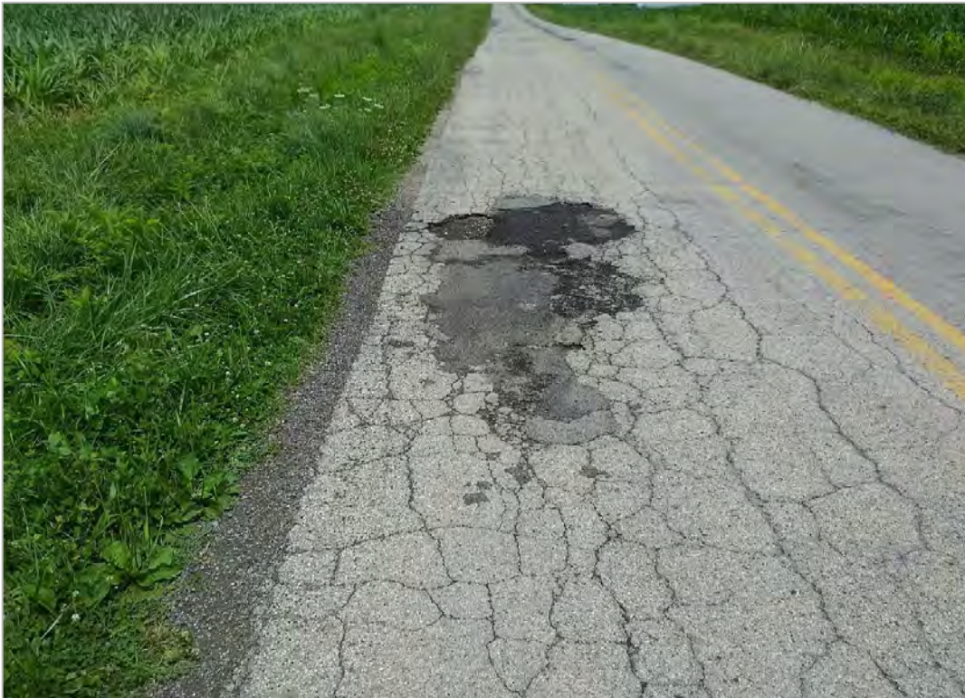
PHOTO 11: Pavement distress (pothole) on Lower Twin Road, looking east.
