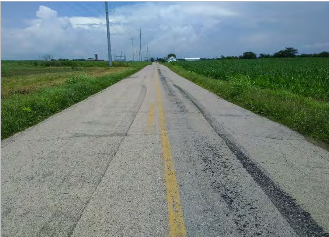
PHOTO 10: Pavement distress (cracked and depressed pavement) over culvert on Lower Twin Road, looking east.
