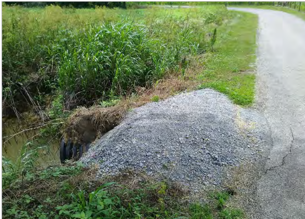
PHOTO 22: Embankment erosion at culvert on Rolfe Road, looking west.
