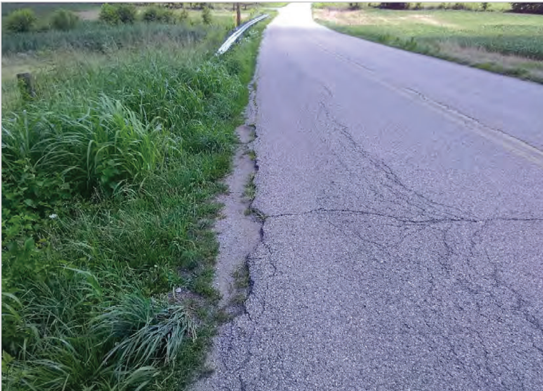
PHOTO 36: Pavement distress (edge failure) on Rapid Forge Road, looking south.
