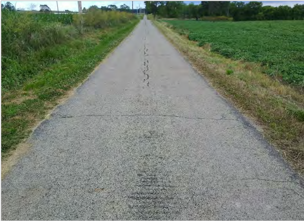
PHOTO 25: Pavement distress (cracked pavement) over culvert on Rolfe Road, looking west.
