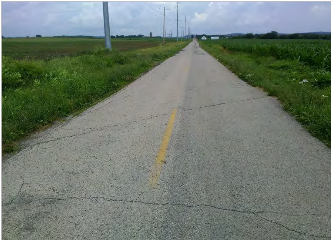
PHOTO 7: Pavement distress (cracked pavement) over culvert on Lower Twin Road, looking east.
