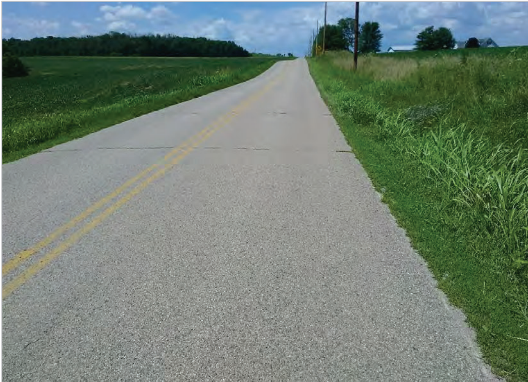
PHOTO 29: Typical pavement distress (transverse cracking) on Rapid Forge Road, looking north.
