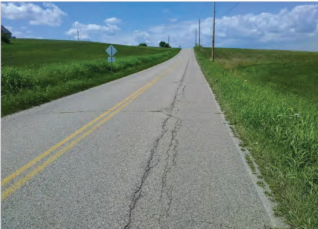
PHOTO 30: Typical pavement distress (transverse and longitudinal cracking) on Rapid Forge Road, looking north.
