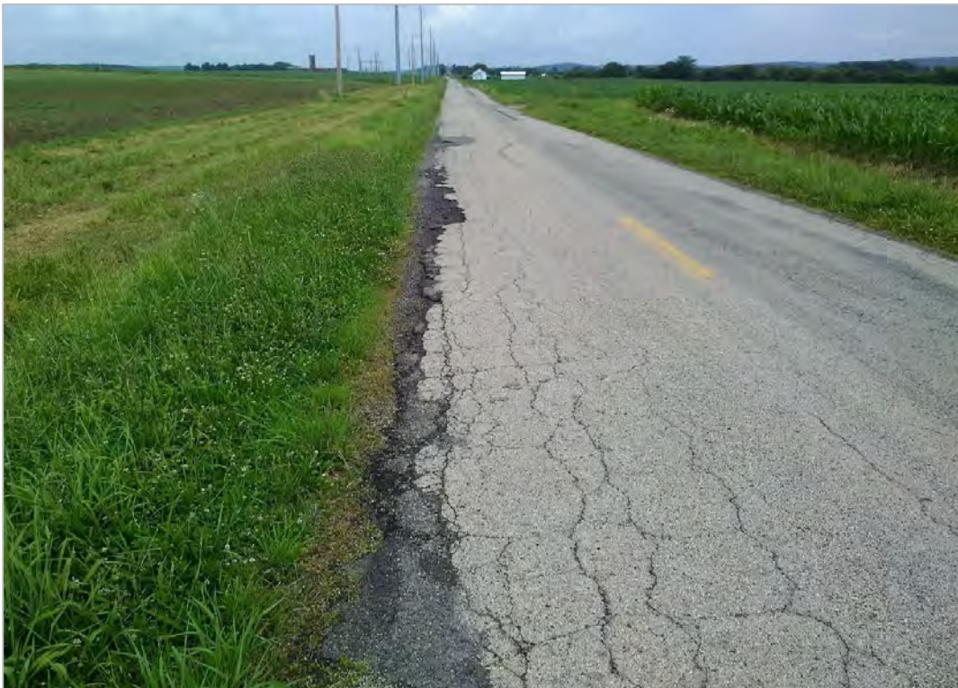
PHOTO 8: Pavement distress (edge failure) on Lower Twin Road, looking east.
