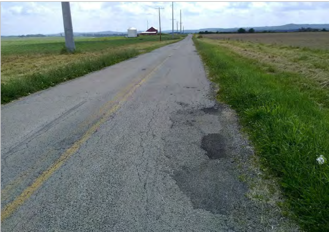
PHOTO 4: Pavement distress (edge deterioration and pothole repair) on Lower Twin Road, looking east.
