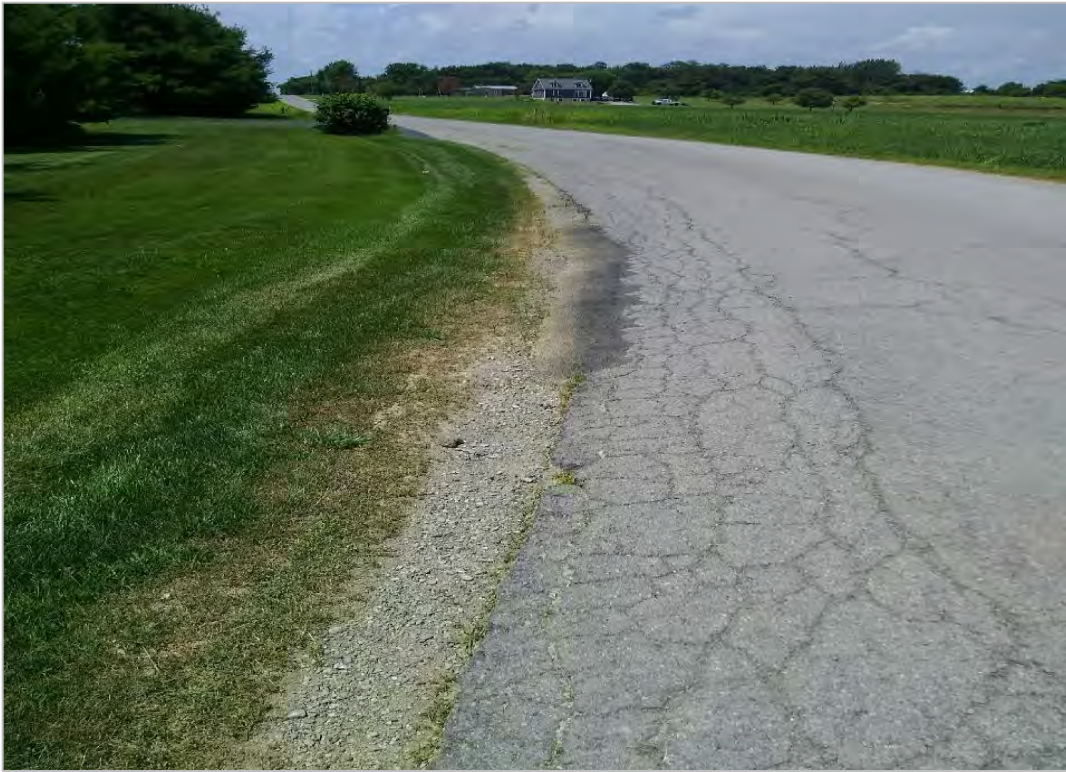
PHOTO 21: Pavement distress (edge deterioration) on Moxley Road, looking west.
