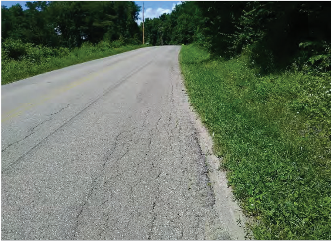
PHOTO 27: Pavement distress (edge deterioration) on Rapid Forge Road, looking north.
