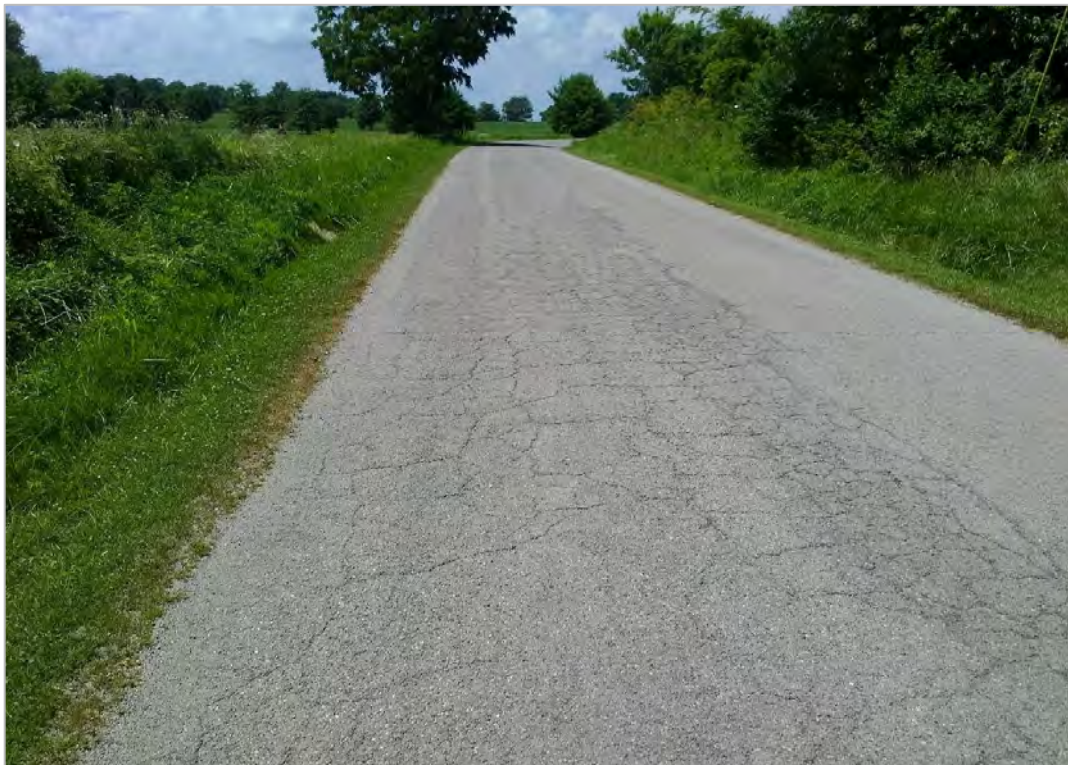
PHOTO 20: Pavement distress (alligator cracking) on Moxley Road, looking west.
