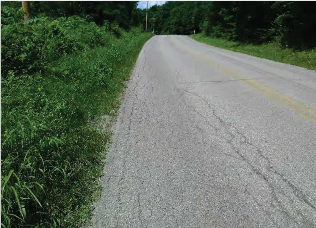
PHOTO 28: Pavement distress (edge deterioration) on Rapid Forge Road, looking north.
