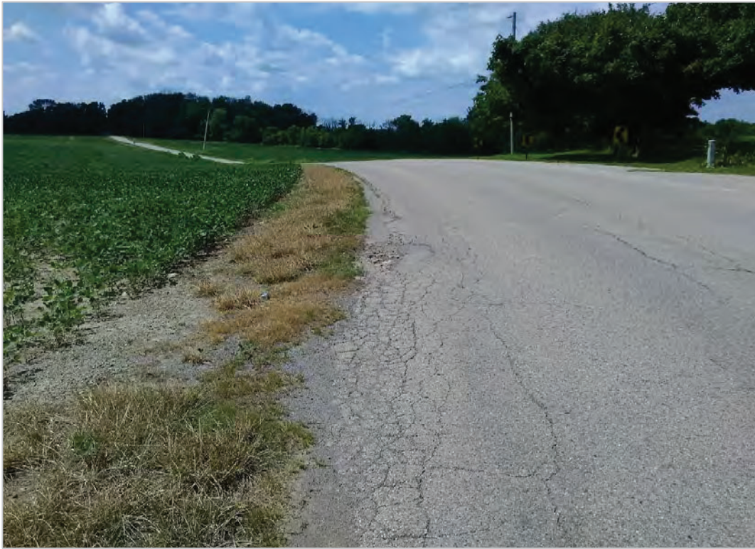
PHOTO 37: Pavement distress (edge failure and pothole) on Rapid Forge Road, looking north.
