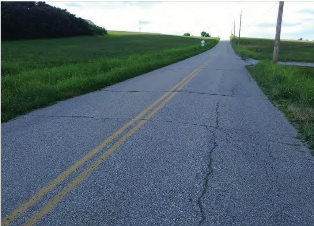
PHOTO 32: Pavement distress (cracked pavement) over culvert on Rapid Forge Road, looking north.
