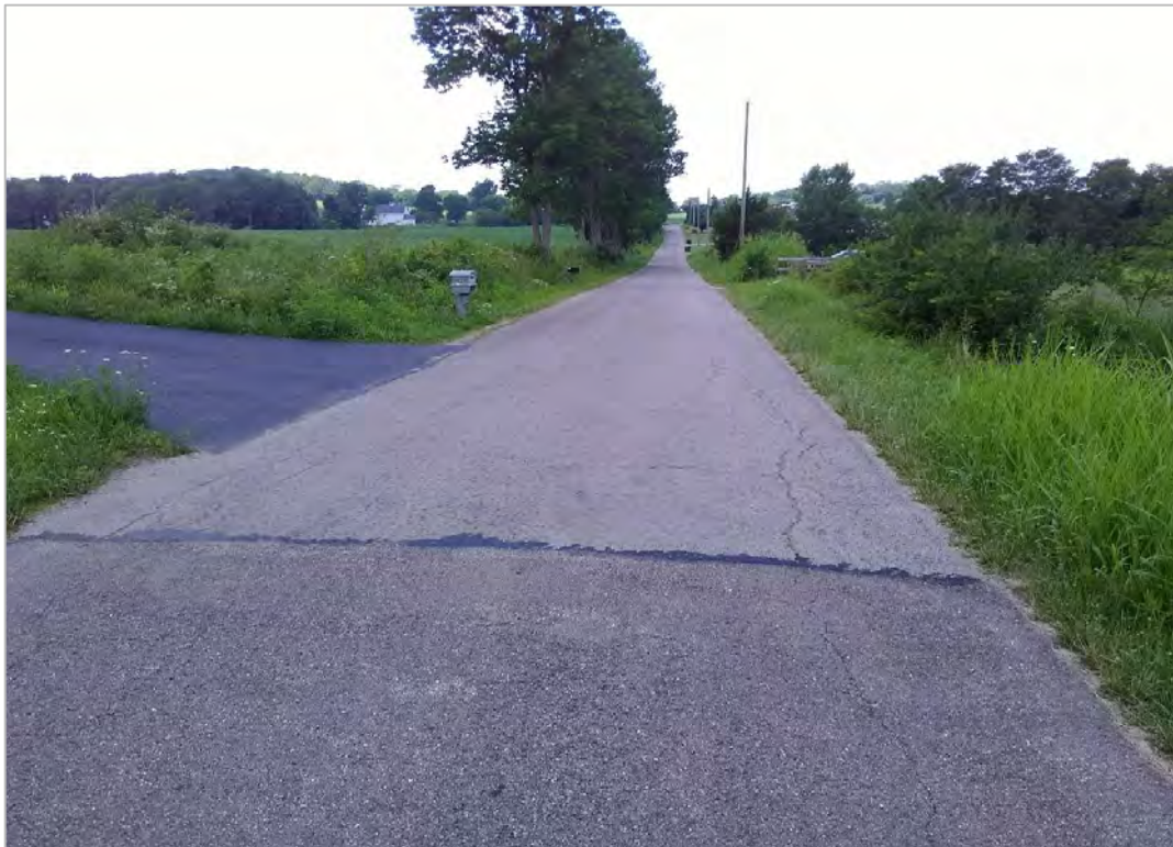
PHOTO 19: View of pavement transition on Moxley Road, looking west. Pavement in good condition east of this location and in fair condition west of this location.
