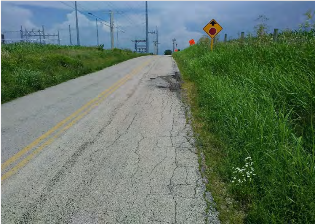
PHOTO 13: Pavement distress (edge failure) on Lower Twin Road, looking east.
