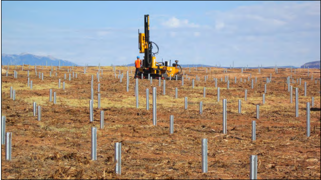
Inset 1. Typical steel support beams for photovoltaic panels and pile-driver during construction (Photo: Clean Energy Collective).
