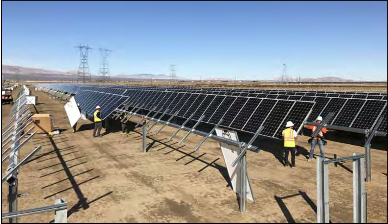
Inset 2. Installation of photovoltaic panel array on steel support beams (Photo: PV Magazine).
