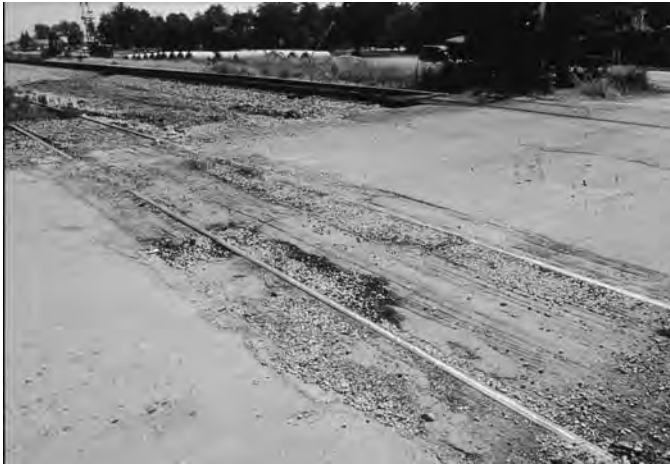
FIG. X1.40 High-Severity Railroad Crossing
