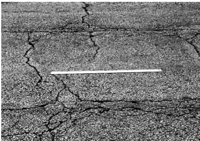
FIG. X1.7 Low-Severity Block Cracking
