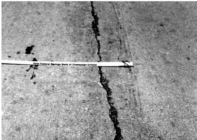
FIG. X2.23 Medium-Severity Linear Cracking
