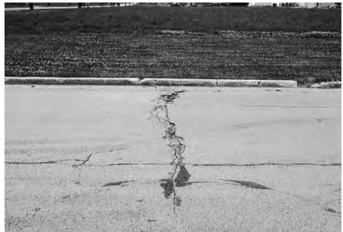
FIG. X1.30 High-Severity Longitudinal and Transverse Cracking
