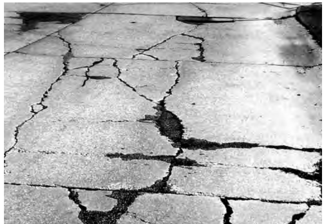
FIG. X2.9 High-Severity Divided Slab
