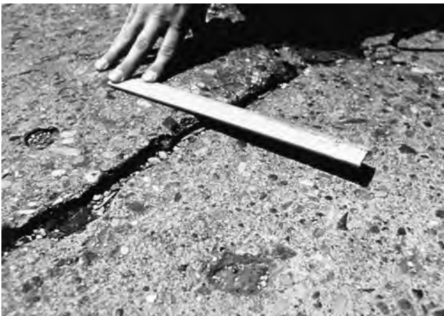
FIG. X2.14 Medium-Severity Faulting
