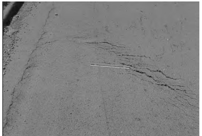
FIG. X1.48 Medium-Severity Slippage Cracking
