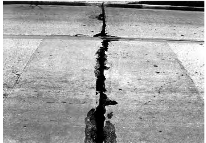
FIG. X2.16 Low-Severity Joint Seal Damage
