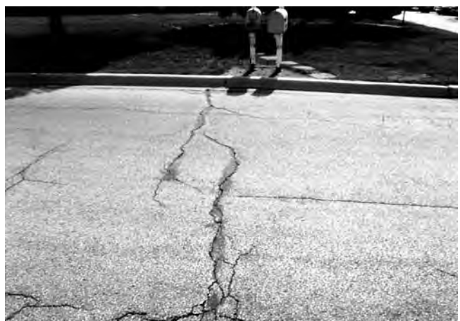
FIG. X1.8 Medium-Severity Block Cracking
