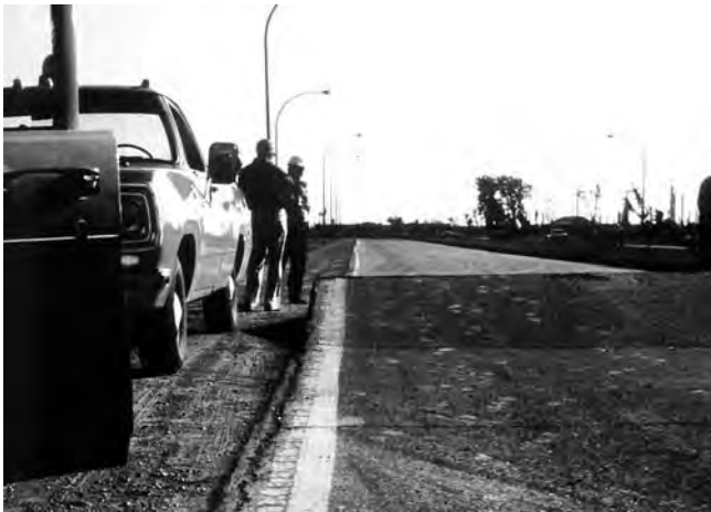
FIG. X2.3 High-Severity Blowup/Buckling
