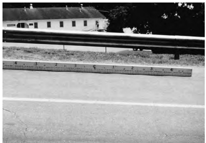
FIG. X1.13 Low-Severity Corrugation
