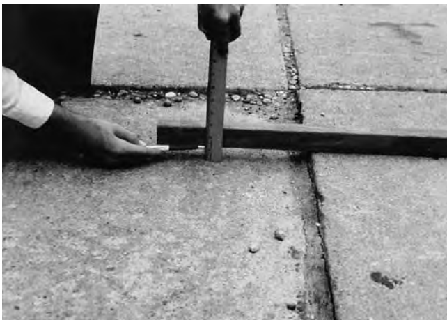
FIG. X2.15 High-Severity Faulting
