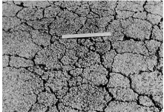
FIG. X1.3 High-Severity Alligator Cracking
