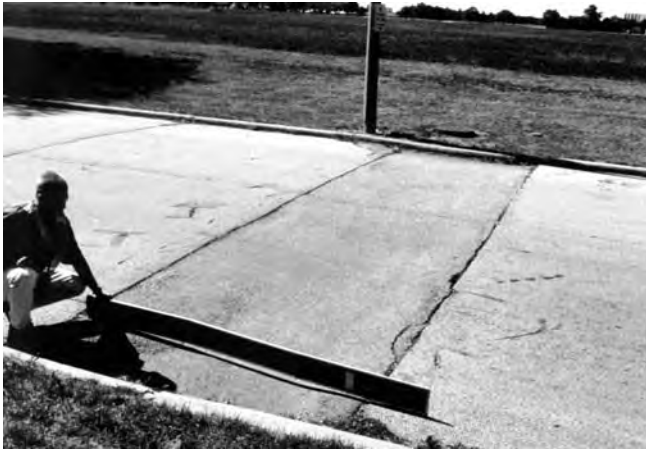
FIG. X1.32 Medium-Severity Patching and Utility Cut Patching
