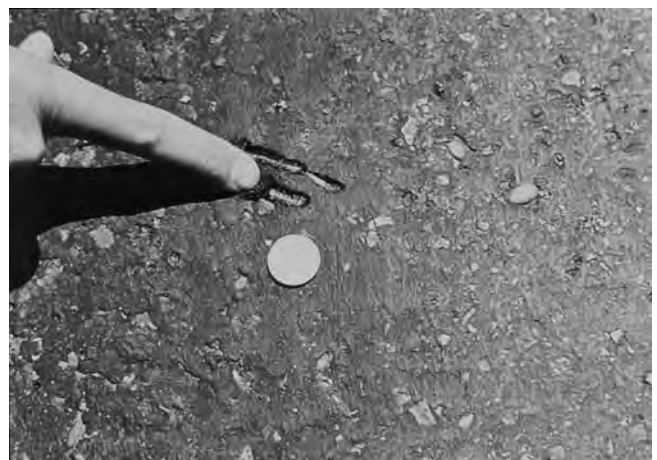
FIG. X1.5 Medium-Severity Bleeding
