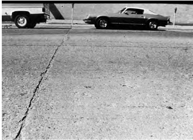
FIG. X2.48 Low-Severity Spalling, Joint
