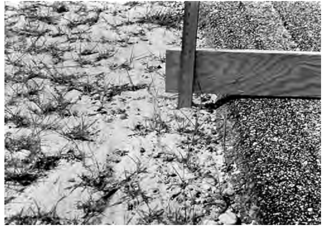
FIG. X1.25 Low-Severity Lane/Shoulder Drop-Off
