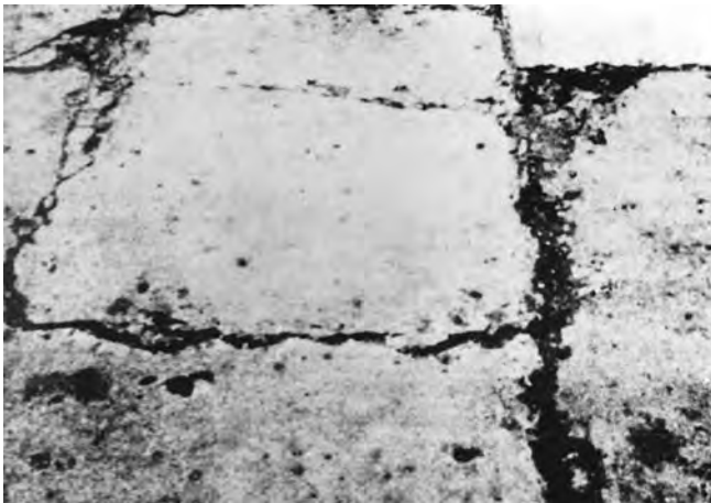
FIG. X2.27 High-Severity Patching, Large and Utility Cuts
