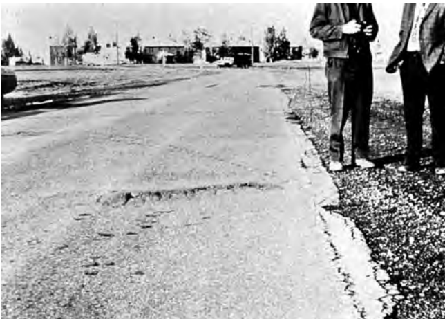
FIG. X1.11 Medium-Severity Bumps and Sags
