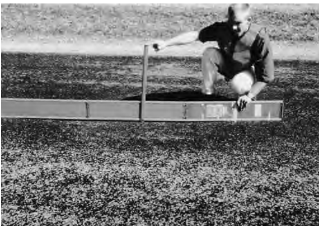
FIG. X1.16 Low-Severity Depression
