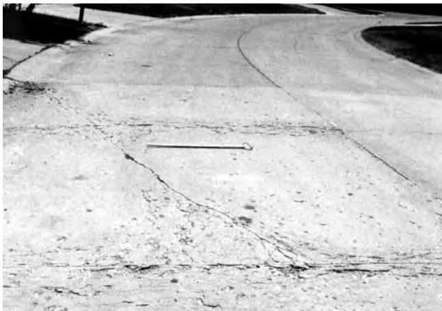
FIG. X2.12 High-Severity Durability Cracking
