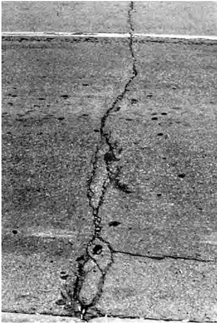
FIG. X1.23 Medium-Severity Joint Reflection Cracking
