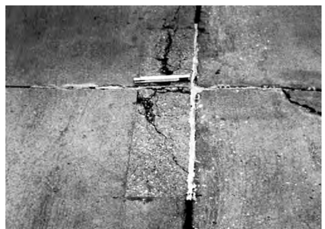
FIG. X2.30 High-Severity Patching, Small
