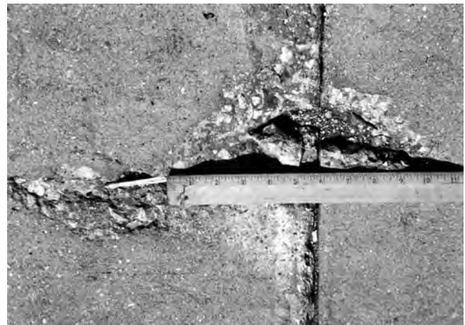
FIG. X2.46 Medium-Severity Spalling, Corner
