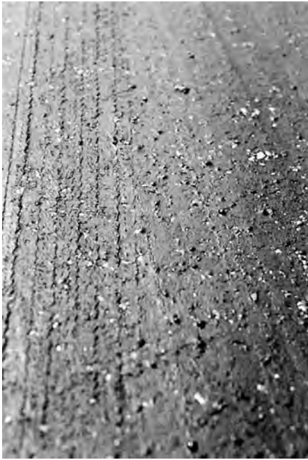
FIG. X1.6 High-Severity Bleeding
