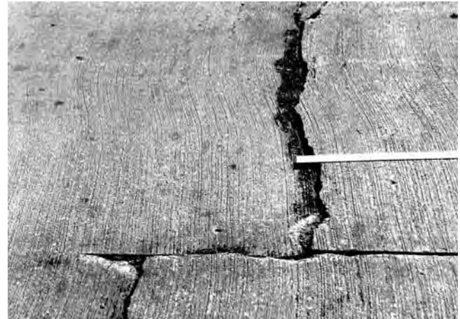
FIG. X2.24 High-Severity Linear Cracking
