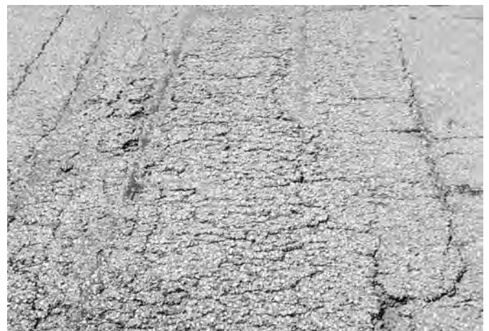
FIG. X1.52 Medium-Severity Weathering and Raveling
