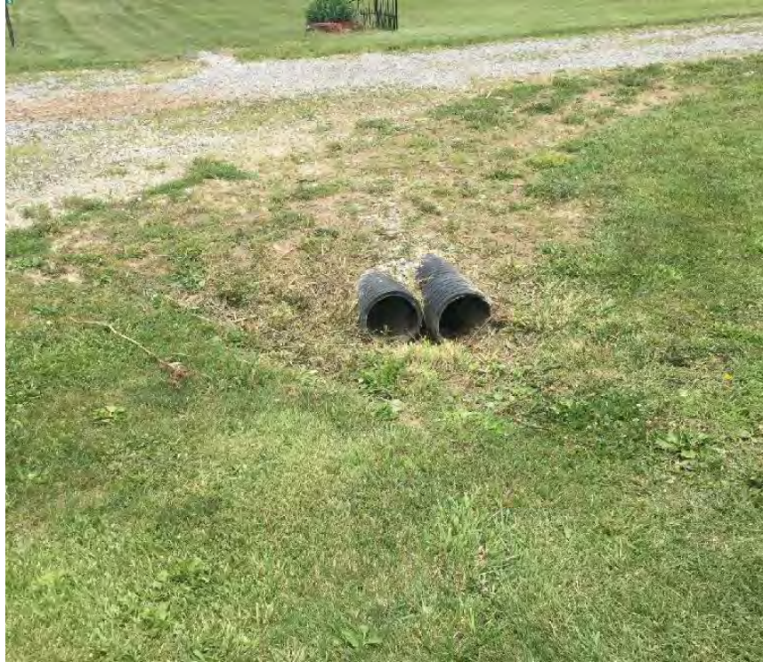
Figure 7-17 CR-75 – Culverts under driveway
