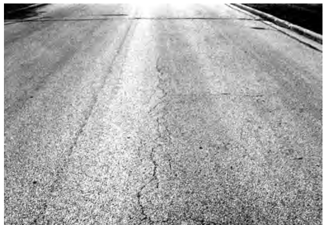
FIG. X1.1 Low-Severity Alligator Cracking
