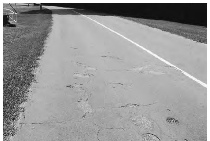
FIG. X1.53 High-Severity Weathering and Raveling
