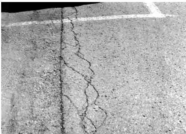
FIG. X1.20 Medium-Severity Edge Cracking
