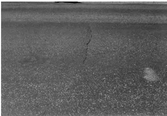
FIG. X1.28 Low-Severity Longitudinal and Transverse Cracking
