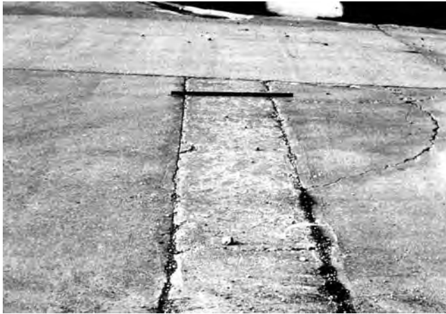
FIG. X2.26 Medium-Severity Patching, Large and Utility Cuts
