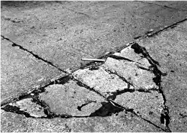
FIG. X2.6 High-Severity Corner Break
