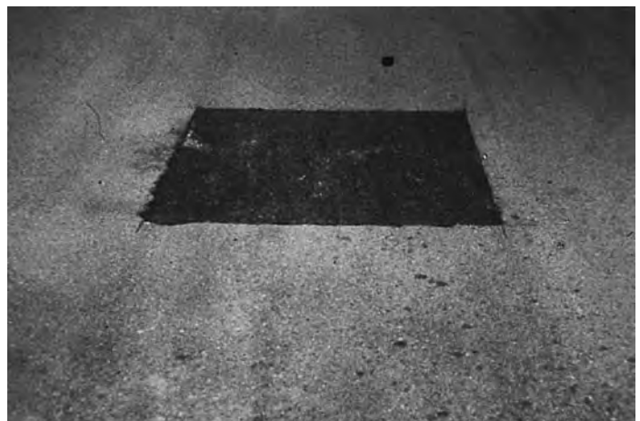
FIG. X1.31 Low-Severity Patching and Utility Cut Patching
