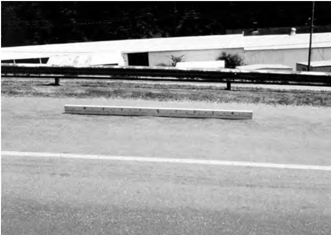
FIG. X1.14 Medium-Severity Corrugation
