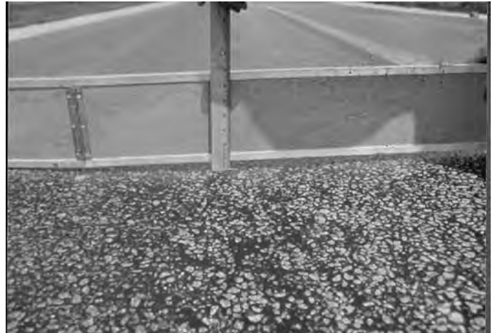
FIG. X1.42 Medium-Severity Rutting
