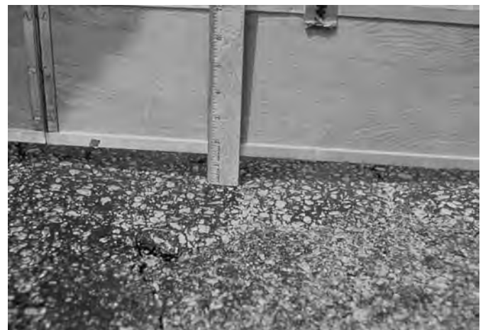
FIG. X1.43 High-Severity Rutting
