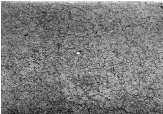
FIG. X2.41 Low-Severity Scaling, Map Cracking, and Craze
