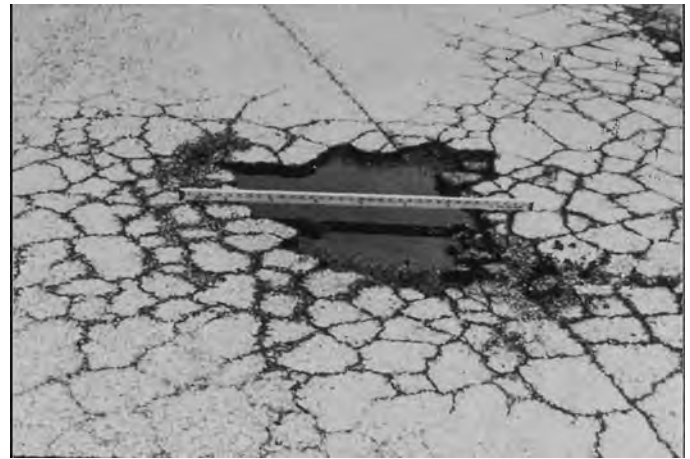
FIG. X1.37 High-Severity Pothole
