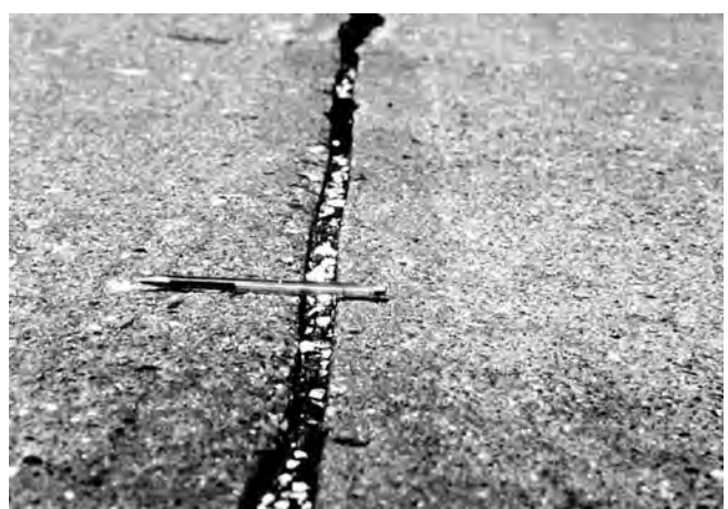
FIG. X2.18 High-Severity Joint Seal Damage
