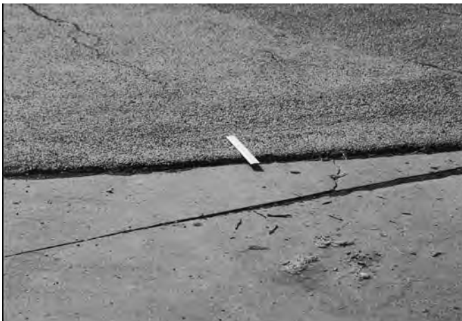
FIG. X1.45 Medium-Severity Shoving
