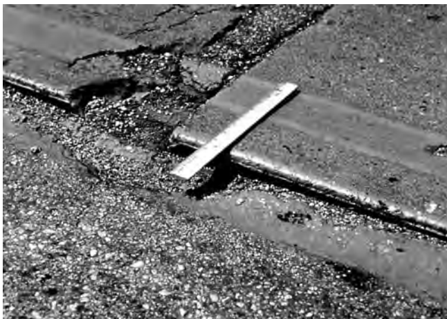
FIG. X2.19 Low-Severity Lane/Shoulder Drop-Off
