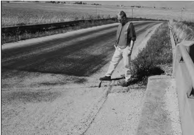
FIG. X1.44 Low-Severity Shoving
