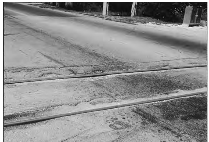
FIG. X1.39 Medium-Severity Railroad Crossing
