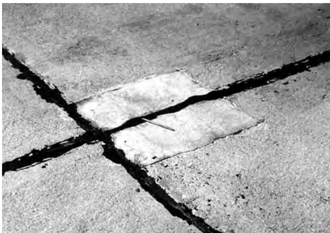
FIG. X2.28 Low-Severity Patching, Small
