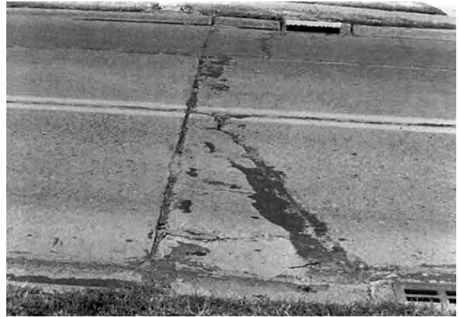
FIG. X2.36 Medium-Severity Punchout
