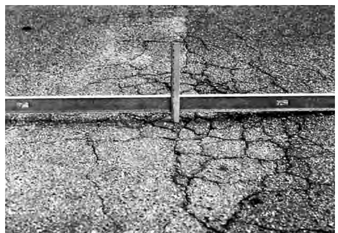
FIG. X1.18 High-Severity Depression
