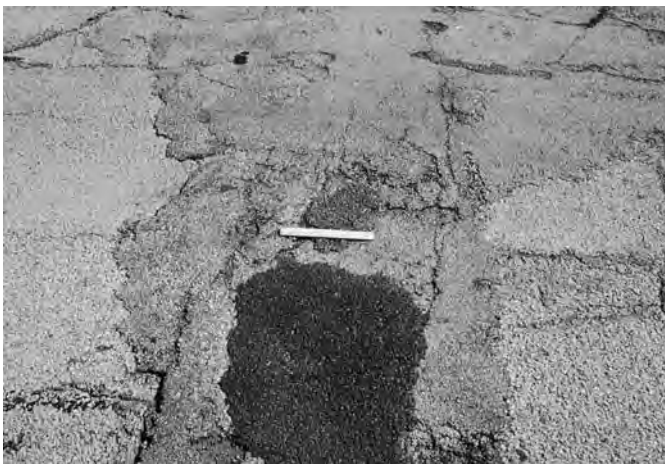
FIG. X1.33 High-Severity Patching and Utility Cut Patching
