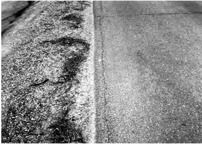
FIG. X1.19 Low-Severity Edge Cracking
