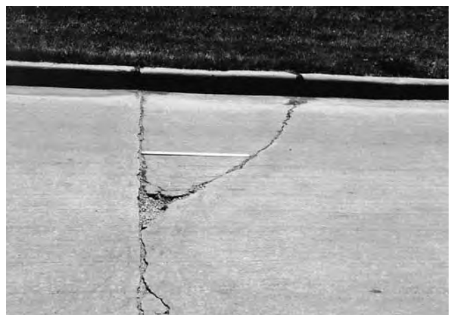
FIG. X2.5 Medium-Severity Corner Break
