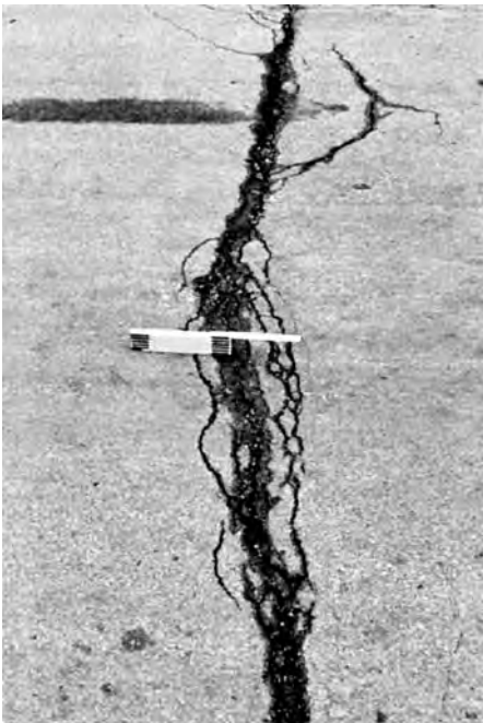
FIG. X1.24 High-Severity Joint Reflection Cracking
