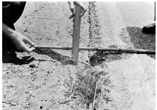
FIG. X1.26 Medium-Severity Lane/Shoulder Drop-Off
