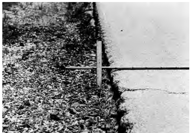
FIG. X1.27 High-Severity Lane/Shoulder Drop-Off
