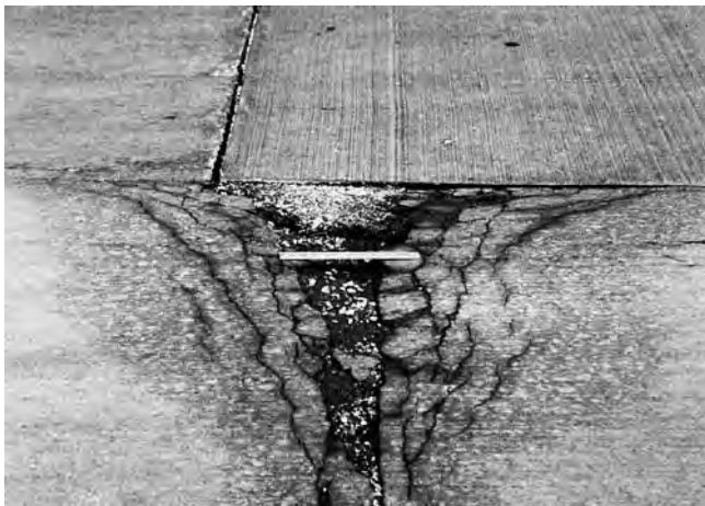
FIG. X2.11 Medium-Severity Durability Cracking
