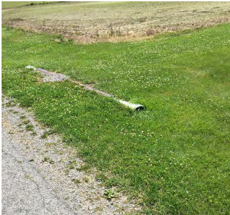
Figure 7-22 CR-75 – Exposed Culvert
