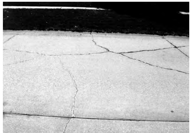
FIG. X2.8 Medium-Severity Divided Slab
