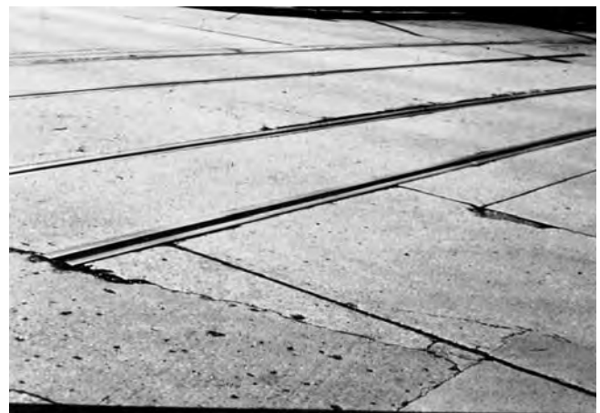
FIG. X2.38 Low-Severity Railroad Crossing
