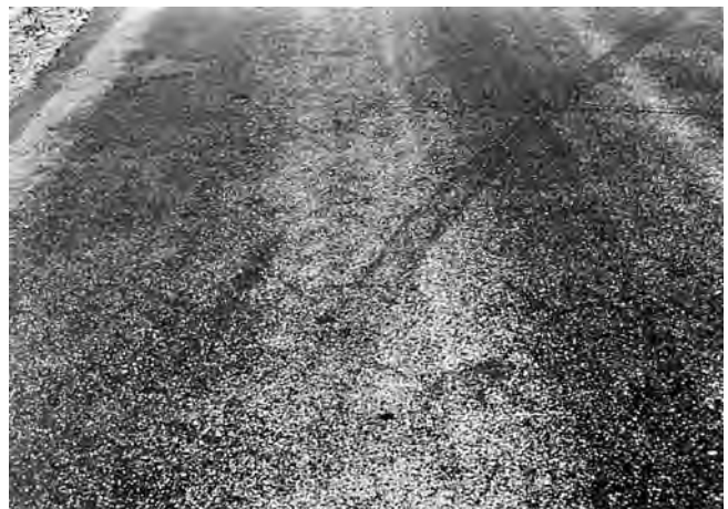
FIG. X1.4 Low-Severity Bleeding
