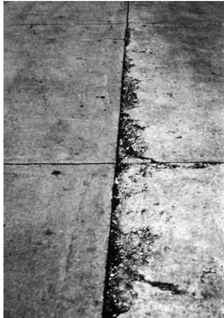
FIG. X2.49 Medium-Severity Spalling, Joint
