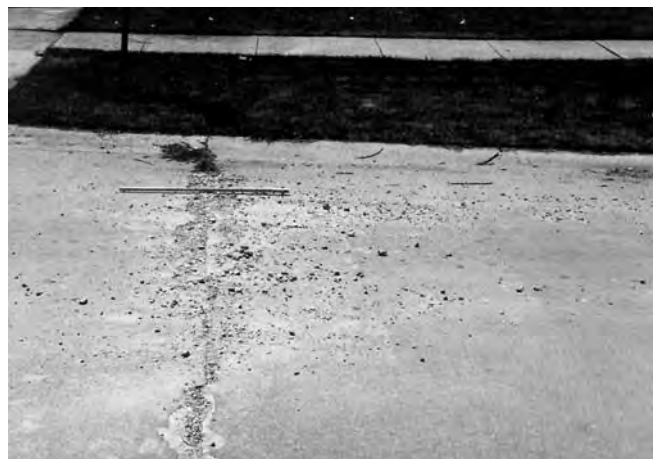
FIG. X2.1 Low Severity Blowup/Buckling
