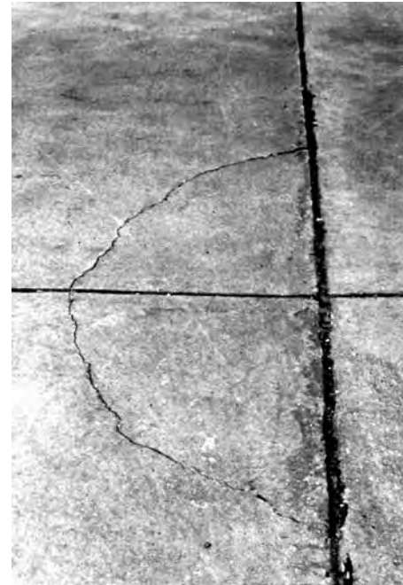
FIG. X2.4 Low-Severity Corner Break
