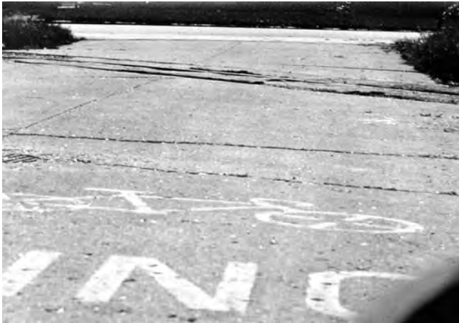
FIG. X2.39 Medium-Severity Railroad Crossing
