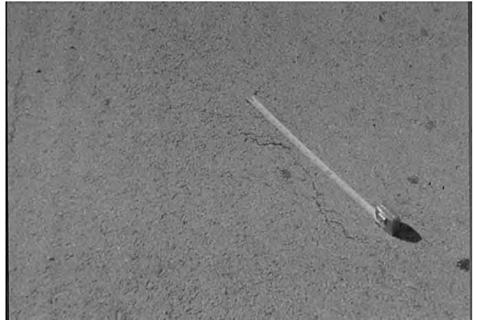
FIG. X1.47 Low-Severity Slippage Cracking
