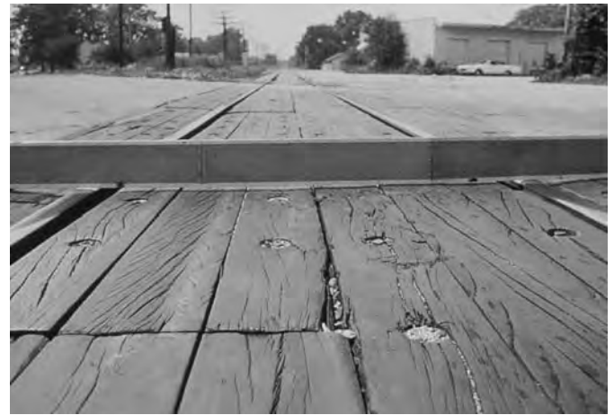
FIG. X1.38 Low-Severity Railroad Crossing
