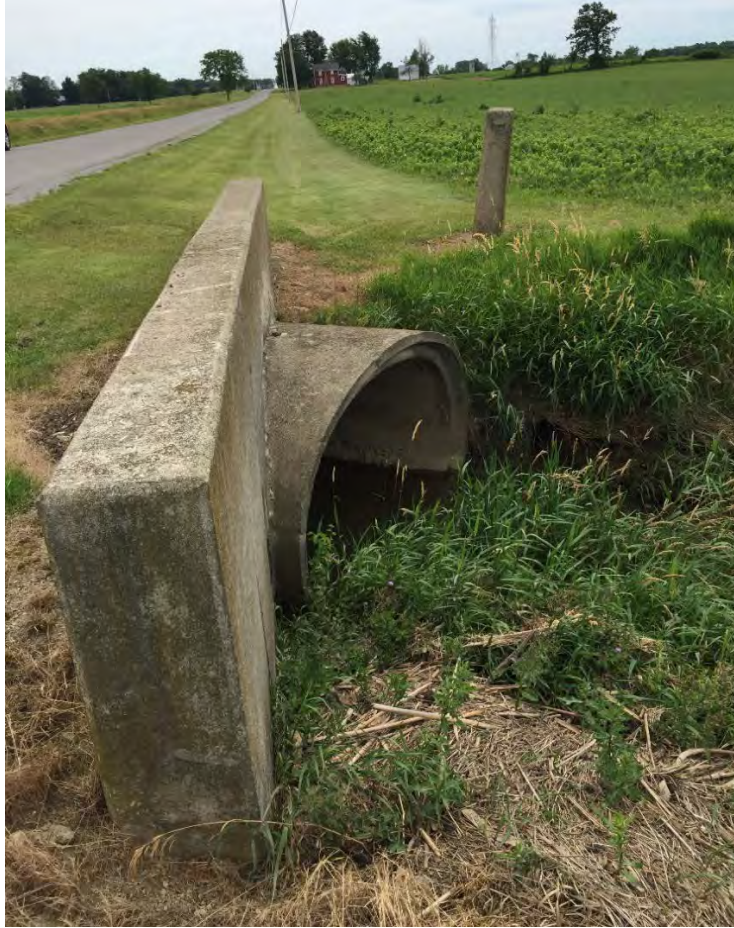
Figure 7-20 CR-75 – 60" RCP Culvert Crossing
