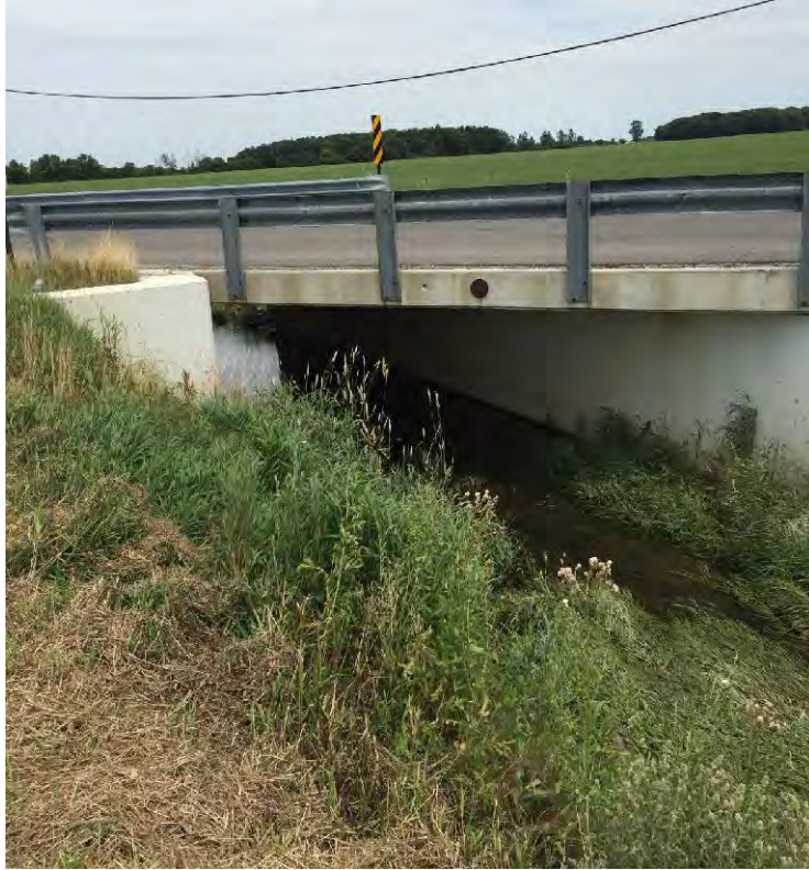
Figure 7-21 CR-75 – Box Culvert Crossing
