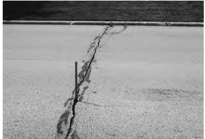
FIG. X1.29 Medium-Severity Longitudinal and Transverse Cracking
