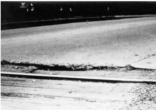
FIG. X2.40 High-Severity Railroad Crossing
