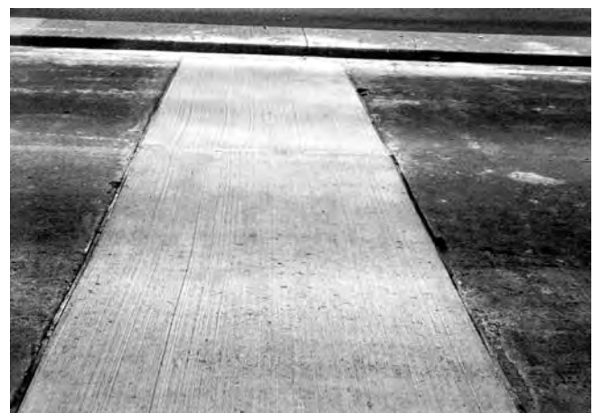
FIG. X2.25 Low-Severity Patching, Large and Utility Cuts
