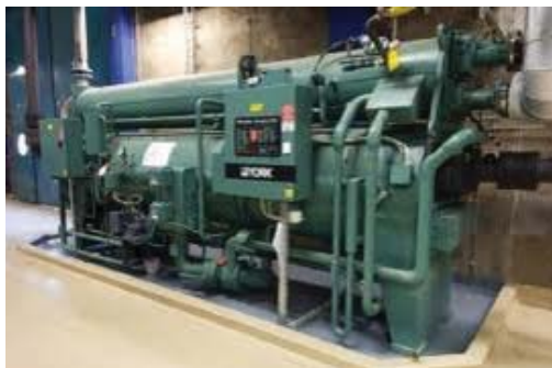
Absorption Chillers University of Lund DES, Sweden
