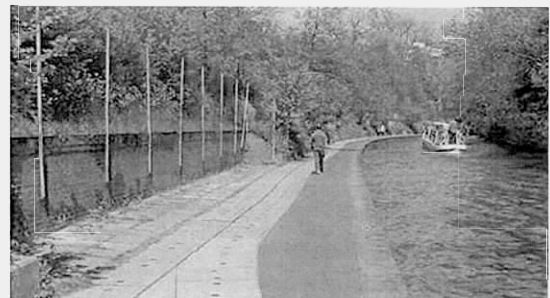
275kV cables installed in surface troughs along tow path
