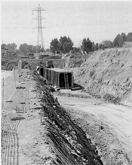
Cut and cover tunnel installation in mainland Europe
