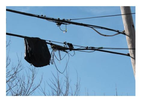
3. This photo from Emery Road, Warrensville Heights, OH shows unsecured cable. The cable should be secured to the utility pole. The wind blows the unsecured service cable, damaging the copper inside the wire and causing service issues. In addition, this cable is within reach of passersby, representing a clear violation of the National Electrical Safety Code (NESC)<sup>1</sup> and causing a public safety hazard.
