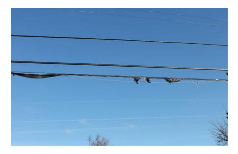
21. This photo from East 2<sup>nd</sup> Street, Girard, OH shows a severely damaged splice terminal. The terminal's protective case is hanging open, leaving wires exposed to weather and animals. Damaged wires cause service outages.
