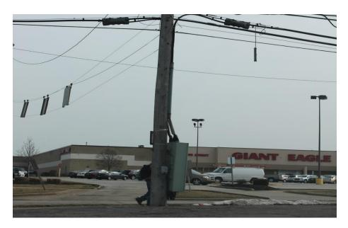
9. This photo from East 135<sup>th</sup> Street, Garfield Heights, OH shows a severely damaged splice box. The box's protective case has deteriorated, leaving wires exposed to weather and animals. Damaged wires cause service outages.
