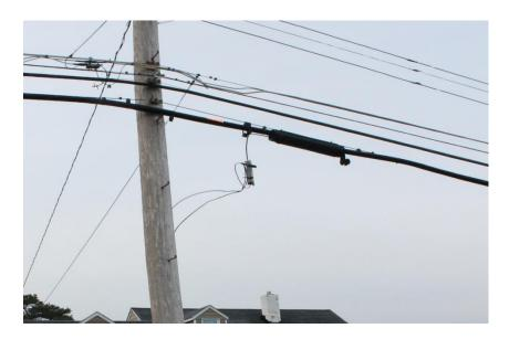
11. This photo from West 48<sup>th</sup> Street, Cleveland, OH shows a badly damaged cable. Instead of replacing the cable, AT&T installed multiple splice boxes on the cable. Each splice box covers a portion of damaged or defective cable. AT&T also used thin drop wires to bypass sections of bad cable. Each of the numerous thin wires would have been installed in response to a separate customer complaint.
