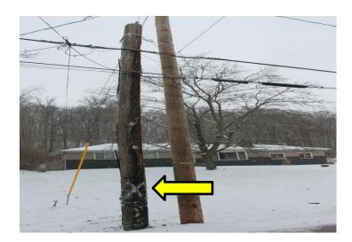
23. This photo from Route 82, Brecksville, OH shows a double-pole. The old pole (right, with a white spray-painted X) with only AT&T equipment attached to it is tied to the new pole with rope to prevent it from falling (yellow arrow). AT&T has not moved its facilities to the new utility pole. As a result, AT&T's equipment remains connected to old, deteriorating poles, causing potential service and safety concerns.
