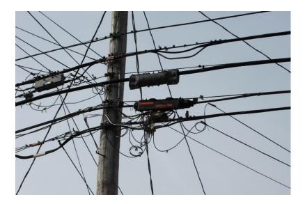
10. This photo from Evelyn Drive, Seven Hills, OH shows an unsecured terminal hanging from service wires. The terminal should be secured to the pole. The terminal can fill with water, deteriorating wires and leading to service issues. In addition, a hanging terminal presents a public safety hazard.
