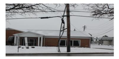
4. This photo from North Linden Lane, Parma, OH shows a double-pole. The old pole (right, with a white spray-painted X) with only AT&T equipment attached to it is tied to the new pole with rope (yellow arrow) to prevent it from falling. AT&T has not moved its facilities to the new utility pole. As a result, AT&T's equipment remains connected to an old, deteriorating pole, causing potential service and safety concerns.
