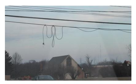
15. This photo from York Road, North Royalton, OH shows a damaged splice wrapped in a makeshift, black plastic covering. Substandard coverings such as this deteriorate rapidly and fail to provide adequate protection. Once the wrap deteriorates, wires are exposed to weather and animals. Damaged wires cause service outages.
