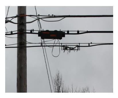
17. This photo from Emery Road, Chagrin Falls, OH shows a damaged splice wrapped in a makeshift, black plastic covering. As noted, substandard coverings such as this deteriorate rapidly and fail to provide adequate protection. Once the wrap deteriorates, wires are exposed to weather and animals. Damaged wires cause service outages.
