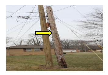
19. This photo from South Thomas Road, Tallmadge Road, OH shows a hanging pole, or a double-pole that has been cut before AT&T moved its facilities to the new pole. The old utility pole was cut with AT&T's terminal still attached to it. Left dangling, the old pole strains the cables and endangers the public. It is a service, worker, and public safety concern.
