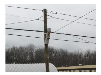
20. This photo from West 2<sup>nd</sup> Street, Girard, OH shows a severely damaged cable. Some remnants of a black plastic cover remain. The cable is damaged, leaving wires exposed to weather and animals. Damaged wires cause service outages.
