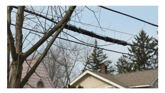
8. This photo from Warrensville Center Road, Maple Heights, OH shows an unsecured terminal hanging from service wires. The terminal should be secured to the pole. The terminal can fill with water, deteriorating wires and leading to service issues. In addition, a hanging terminal presents a public safety hazard to passersby.
