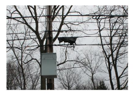
16. This photo from Wexford, Parma, OH shows a severely damaged splice terminal. The terminal's protective case is missing, leaving wires exposed to weather and animals. Damaged wires cause service outages.
