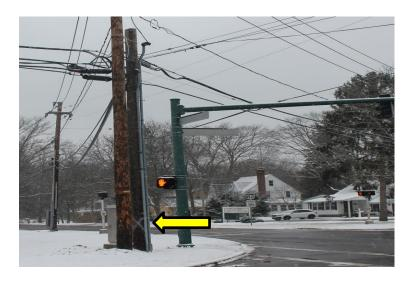
24. This photo from Hillside Street, Cuyahoga Falls, OH shows a badly damaged cable. Instead of replacing the cable, AT&T installed multiple splice boxes on the cable. Each splice box covers a portion of damaged or defective cable. AT&T also used drop wires to bypass sections of bad cable. Each of the numerous thin wires would have been installed in response to a separate customer complaint.
