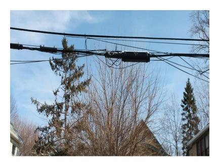
12. This photo from Brown Avenue, Newburgh Heights, OH shows a severely damaged splice terminal. The terminal's protective case is hanging open, leaving wires exposed to weather and animals. Damaged wires cause service outages.
