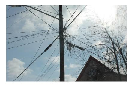
13. This photo from Forest Drive, Pepper Pike, OH shows an exposed terminal (yellow arrow). The terminal's protective case is hanging open, leaving wires exposed to weather and animals. Damaged wires cause service outages.
