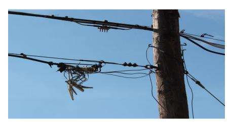
2. This photo from Delaware Avenue, Youngstown, OH shows a severely damaged splice terminal. The terminal's protective case is hanging open, and the black plastic covering meant to protect wires has fallen off, leaving wires exposed to weather and animals. Damaged wires cause service outages.
