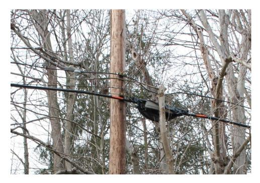
7. This photo from Charles Street, Maple Heights, OH shows a badly damaged cable. Instead of replacing the cable, AT&T attempted to resolve the problem with multiple splices in a span of a few feet on the cable. Each splice box covers a portion of damaged or defective cable.
