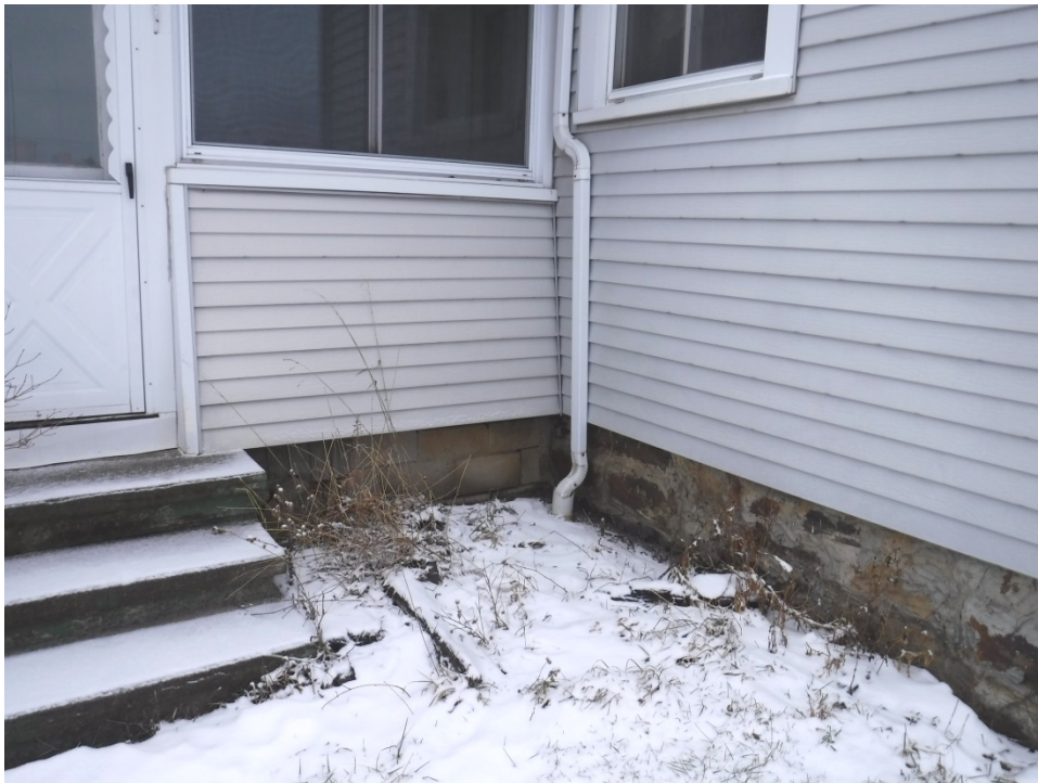
Photo 10. Detail of RIC0093711 foundation, facing northeast Main foundation on right is coursed rubble sandstone, and porch foundation on left is concrete block
