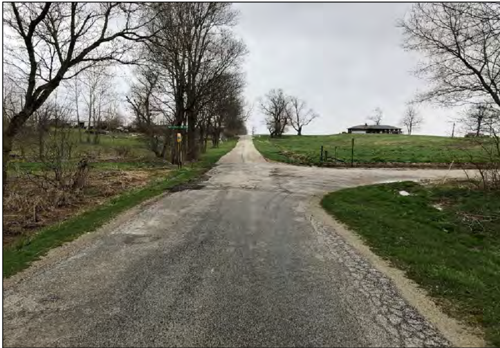
PHOTO 7: Pavement deterioration at intersection of State Line and Paint Creek Four Mile Roads.
