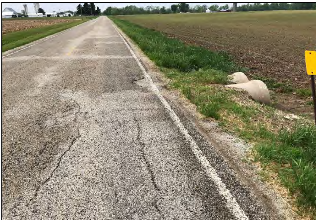
PHOTO 8: Pavement depression over twin RCP culverts on Paint Creek Four Mile Road.
