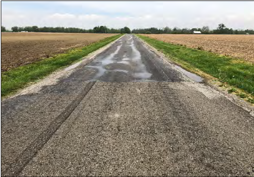
PHOTO 5: Pavement transition from 17 feet wide to 15 feet wide on State Line Road. Note slight rutting and edge cracking on 15-foot section.
