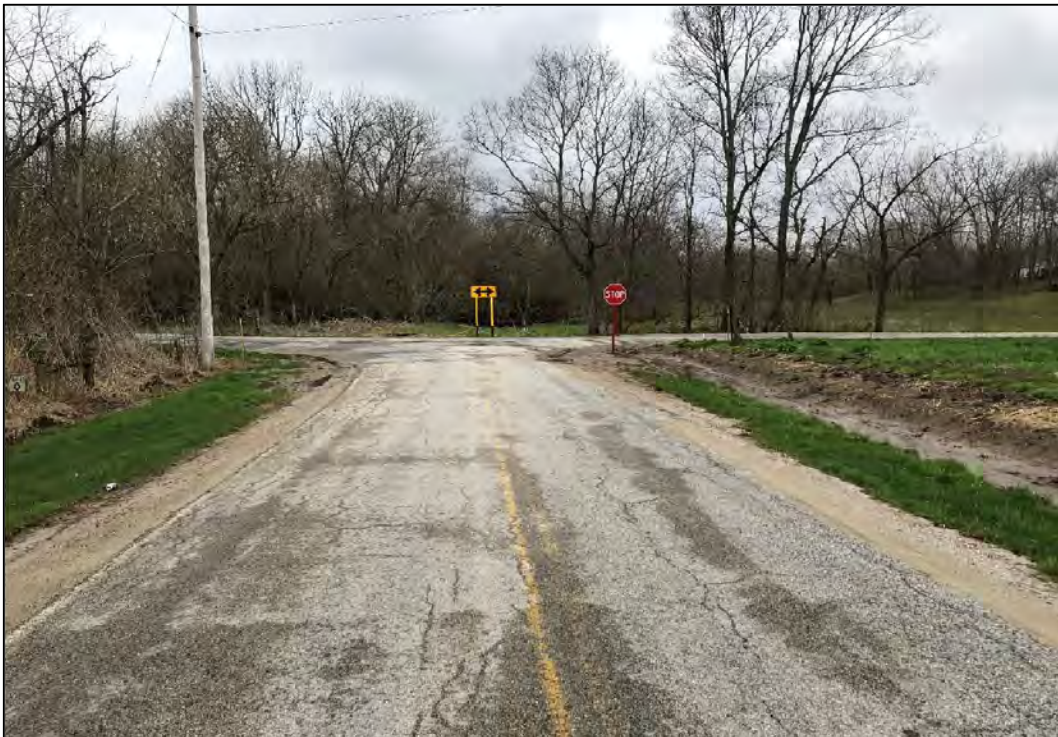
PHOTO 5: Pavement transition from 17 feet wide to 15 feet wide on State Line Road. Note slight rutting and edge cracking on 15-foot section.
