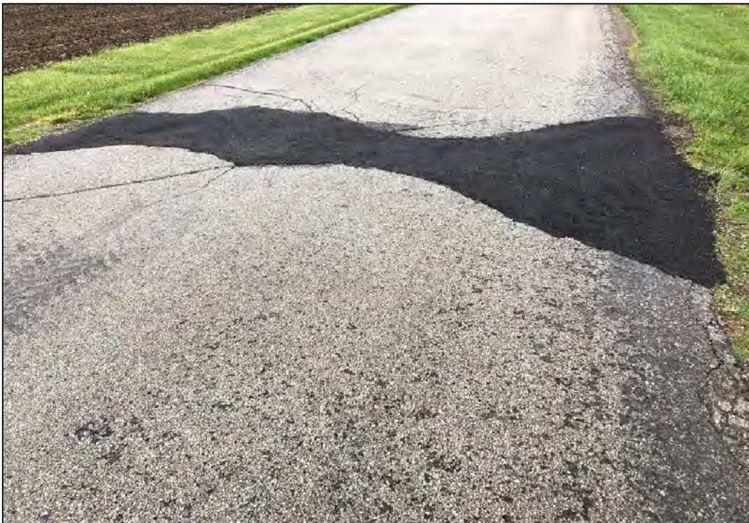
PHOTO 2: Pavement repair on State Line Road just north of State Route 725.
