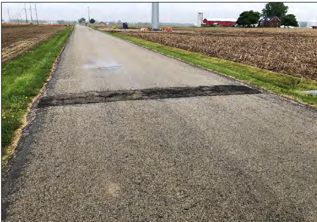
PHOTO 4: Pavement repair on State Line Road over CMP culvert just north of Campbell Road.
