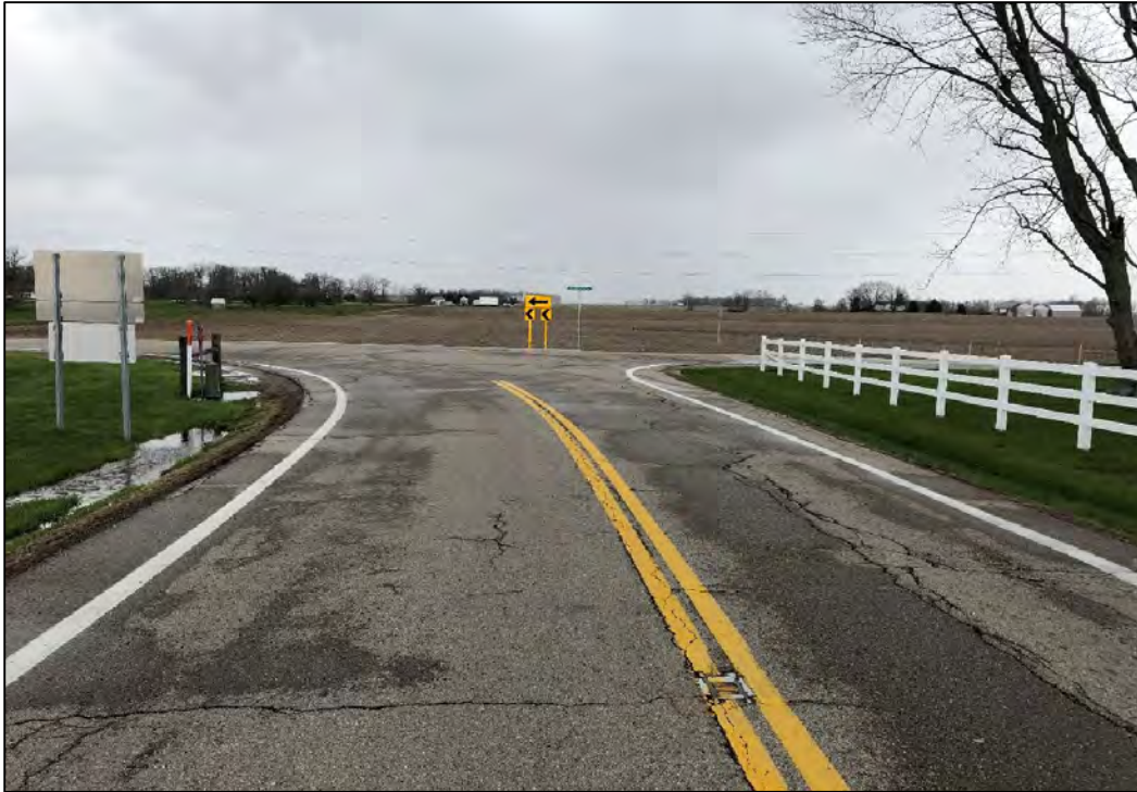
PHOTO 1: View of longitudinal cracking on SR725.
