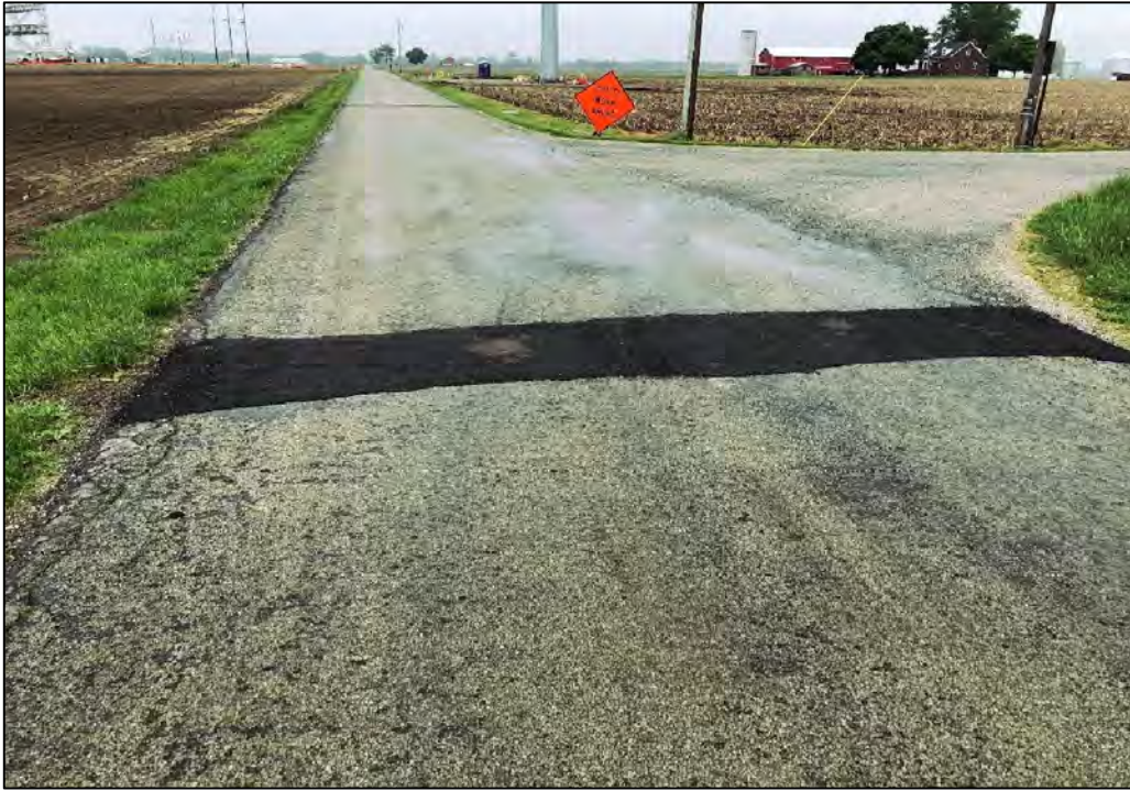
PHOTO 3: Pavement repair on State Line Road over CMP culvert just south of Campbell Road.
