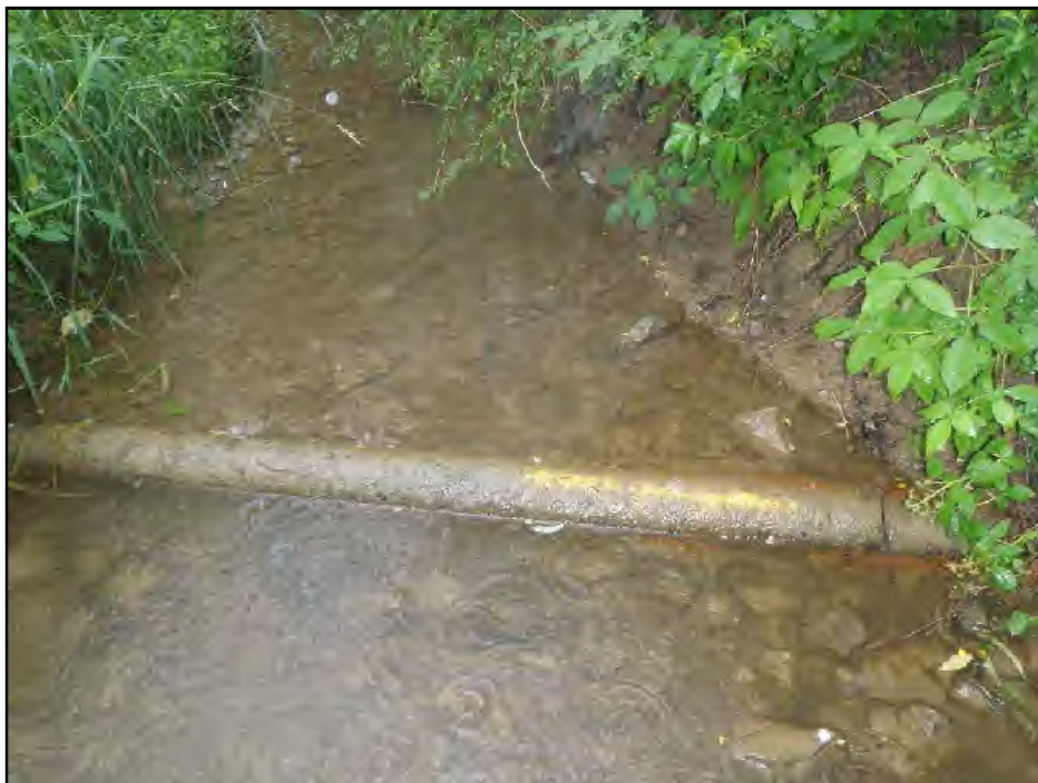
Photograph 4. The existing gas pipeline is exposed within Stream 1.
