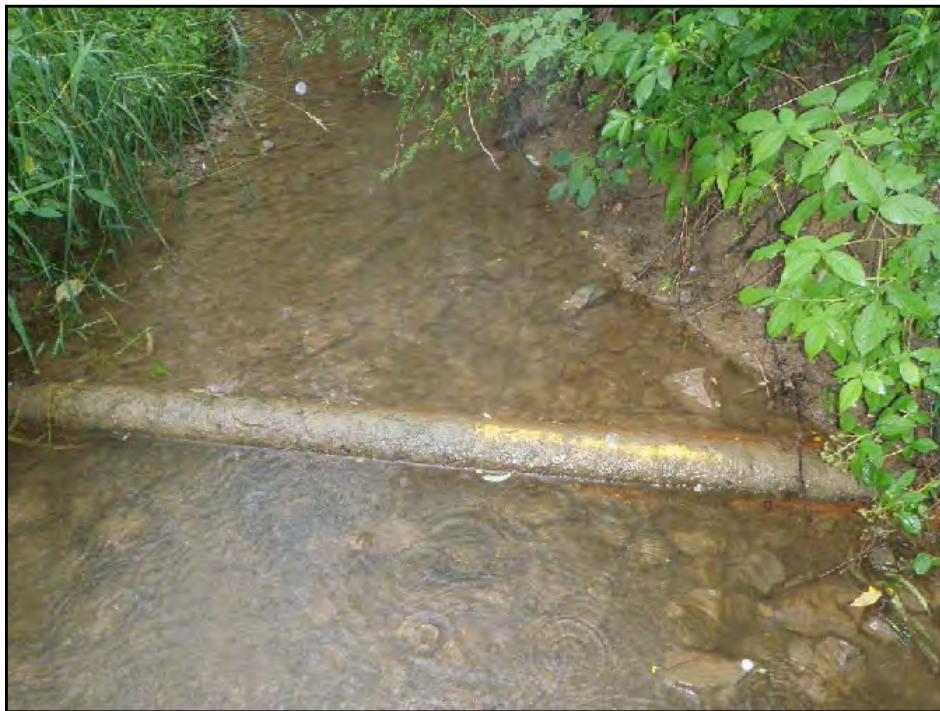
Photograph 6. The gas pipeline is exposed within Stream 1a.
