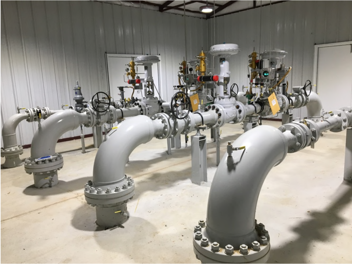
EXAMPLE OF REGULATING STATION
