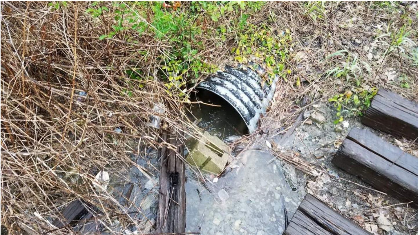
Pearl 016 - 24" CMP Culvert, Plugged - NE QUAD looking Southwest
