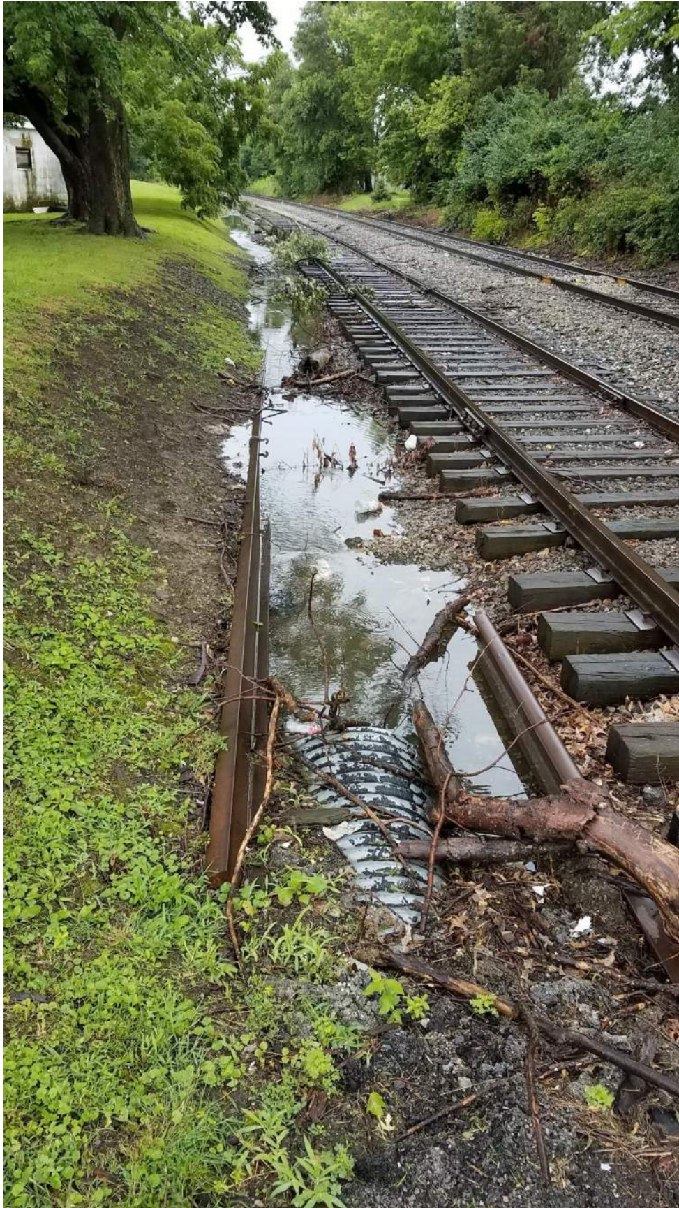
Pearl 019 - 24" CMP Culvert, Plugged - SE QUAD looking Southwest
