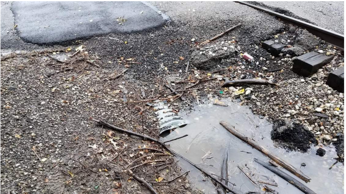
Pearl 008 - 24" CMP Culvert, Plugged - SW QUAD looking Northeast
