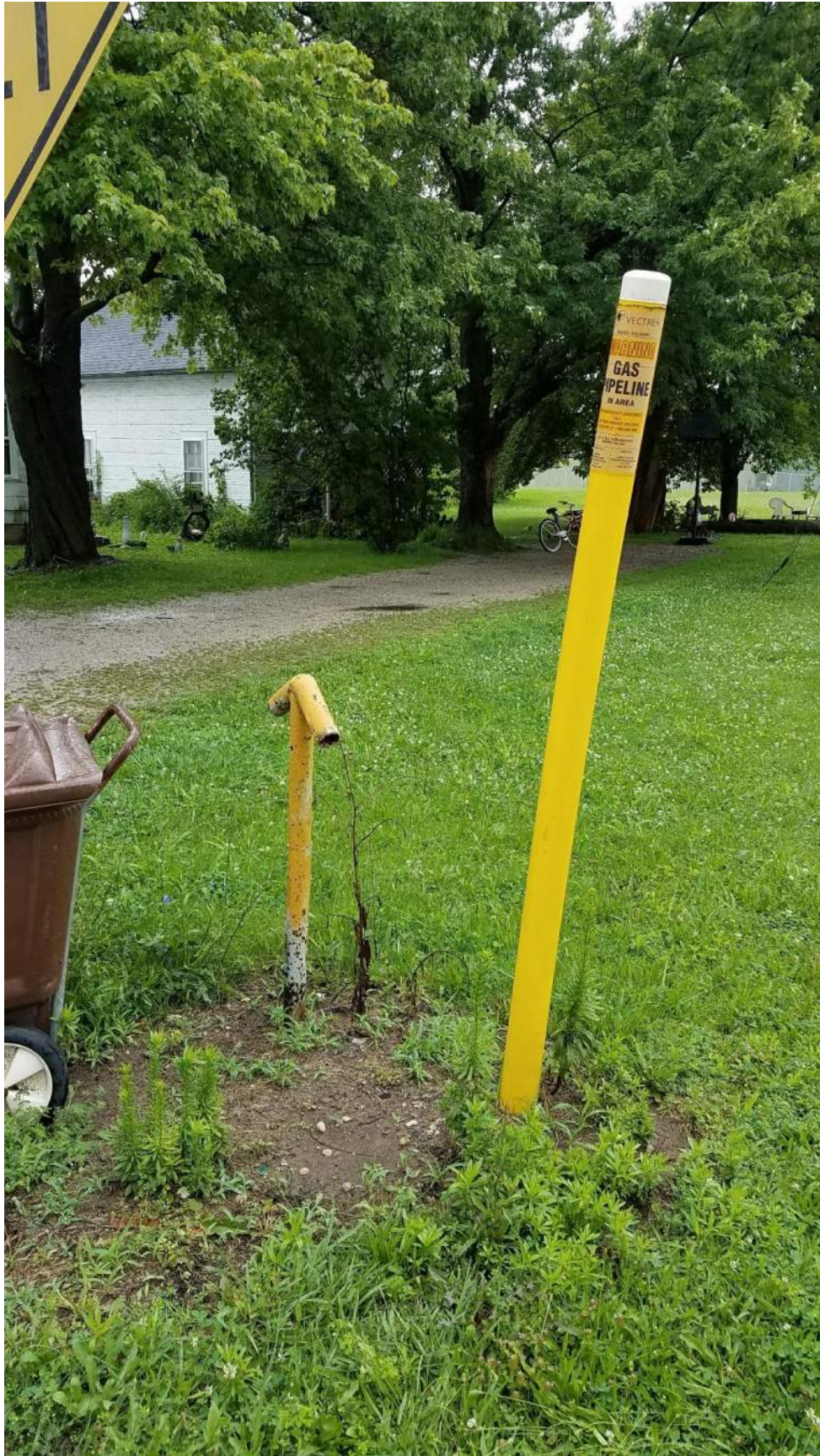
Pearl 011 - Gas Marker and Vent, Perpendicular to Tracks - NW QUAD looking Northwest
