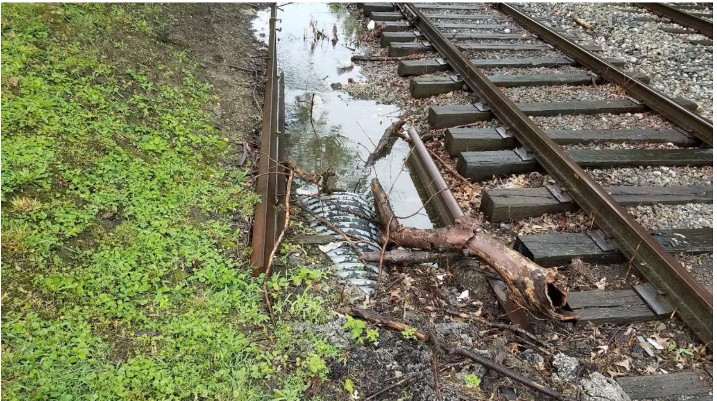
Pearl 018 - 24" CMP Culvert, Plugged - SE QUAD looking Southwest
