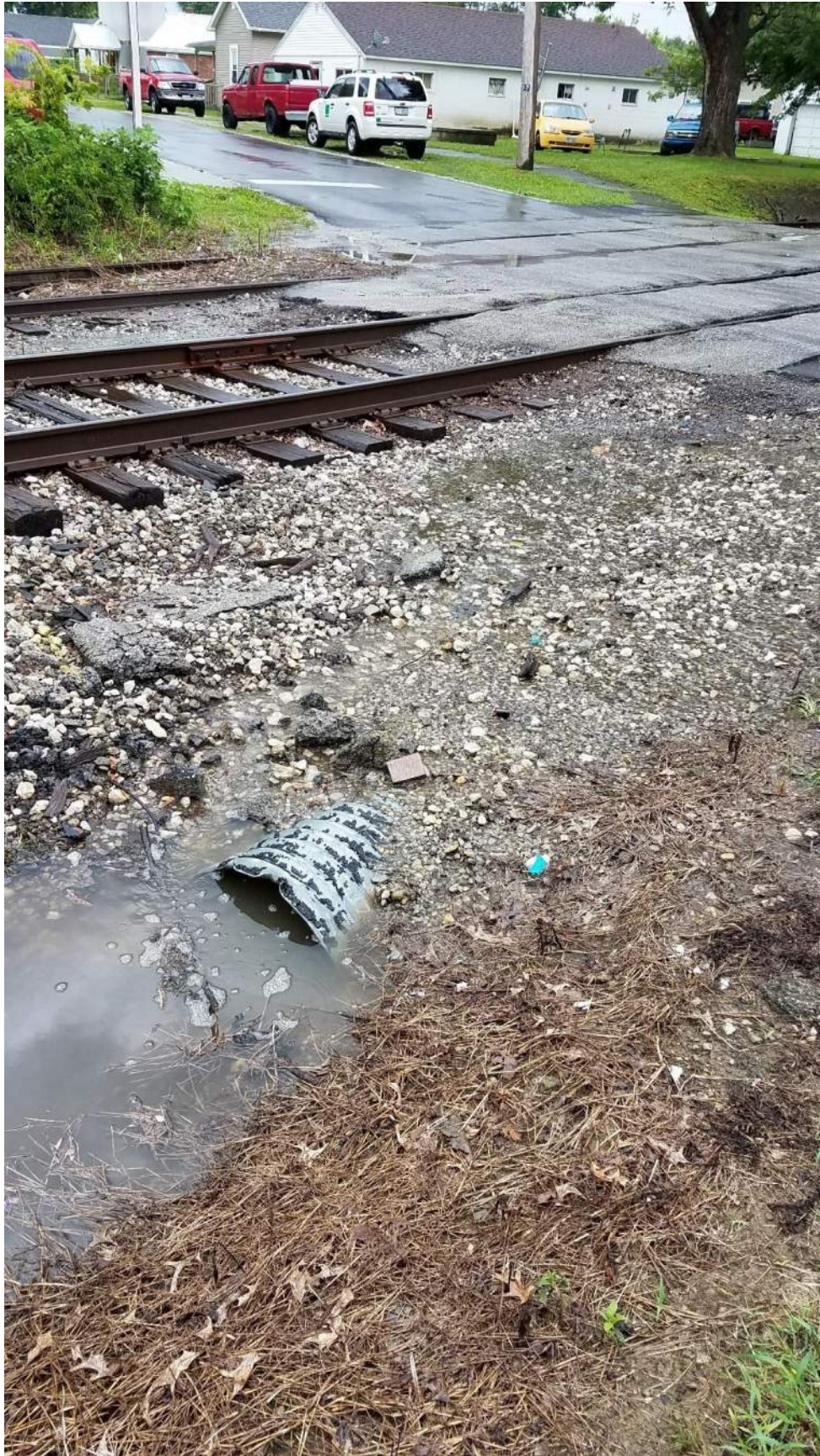
Pearl 009 - 24" CMP Culvert, Plugged - NW QUAD looking South
