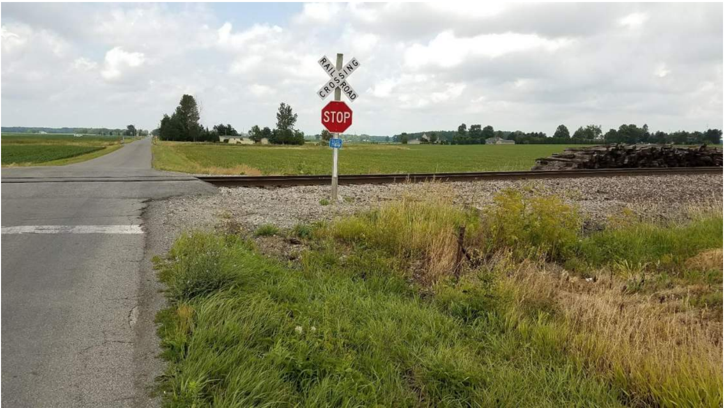
Van Atta Rd 012 - Existing Passive Warning Devices - SE QUAD looking North
