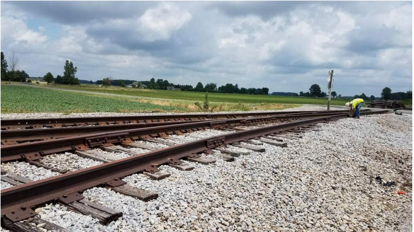
Van Atta Rd 005 - Cooperative Turnout Insulated Joints and Crossing Surface - SW QUAD looking Northeast
