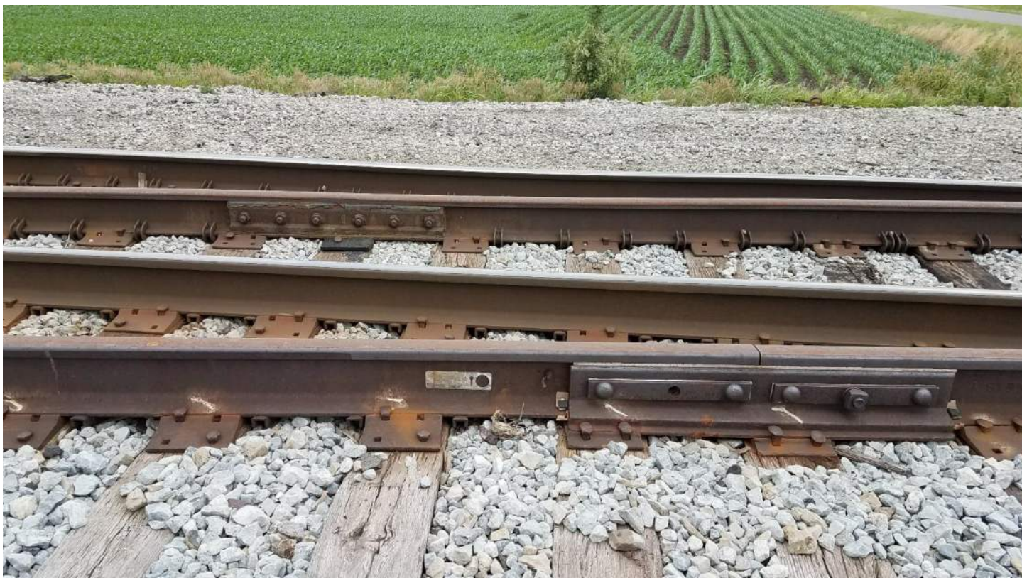
Van Atta Rd 004 - Cooperative Turnout Insulated Joints - SW QUAD looking North
