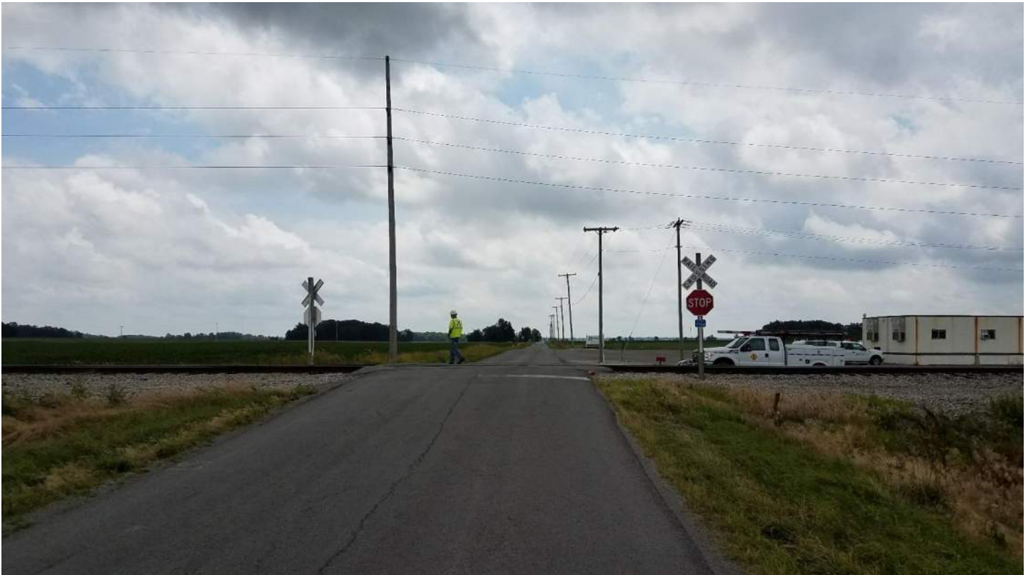
Van Atta Rd 010 - Existing Passive Warning Devices - NW QUAD looking South
