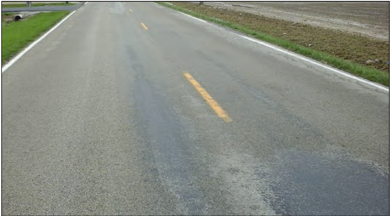
Small asphalt cracking/potholes/touch-ups along road.
