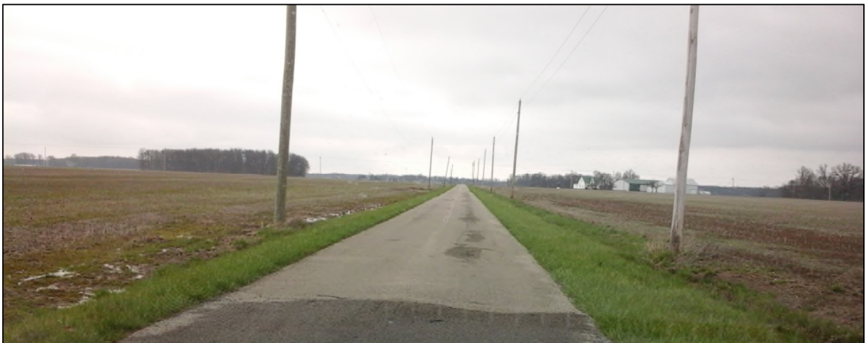
Small Asphalt repair transition stretch.
