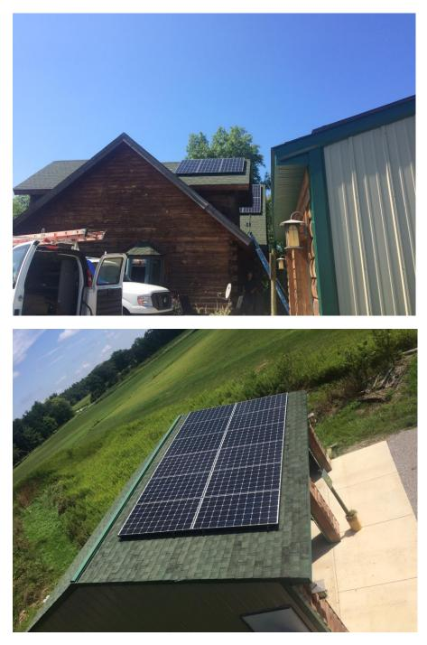
The nameplate capacity of the system is 5.4kW.
