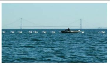
Figure 5-8. Small workboats keep the cable in position
