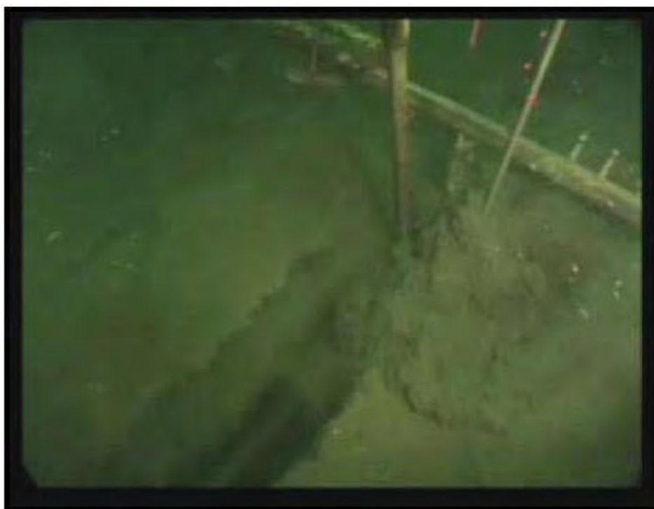
Figure 8-18: Jetting Equipment in Operation
