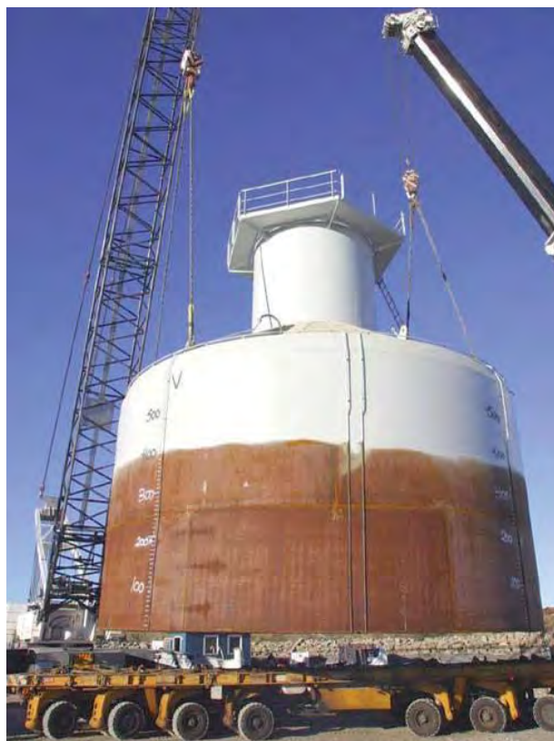
Figure 6-26: Prototype Suction Caisson
