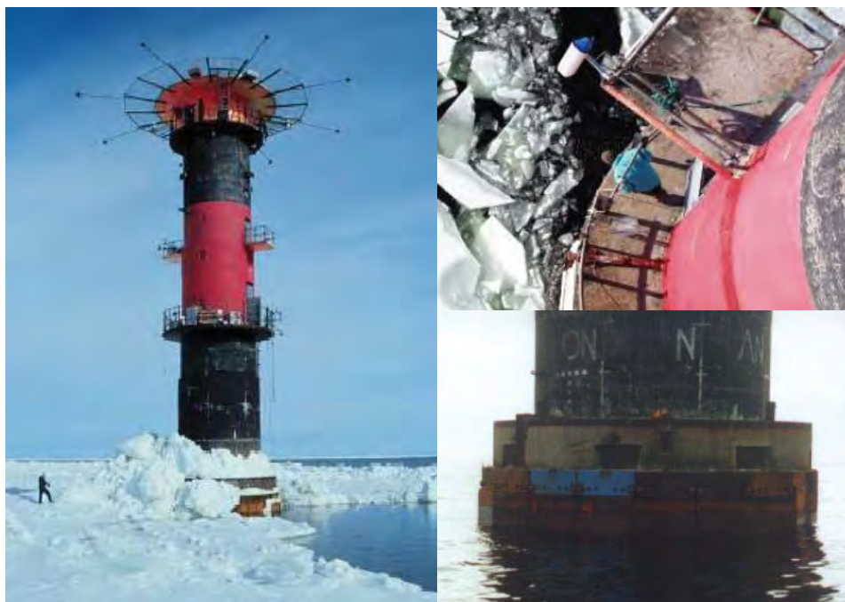
Figure 7-2: Ice Measurements on a Lighthouse in the Swedish Baltic Sea (Project STRICE)
