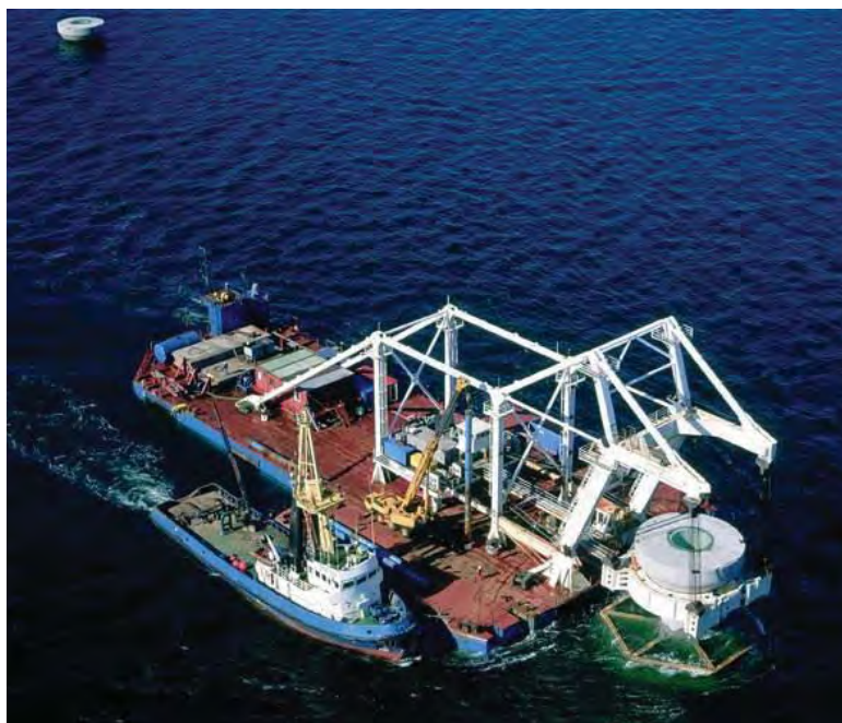
Figure 6-25: Gravity Foundations Being Installed at Nysted, Denmark
