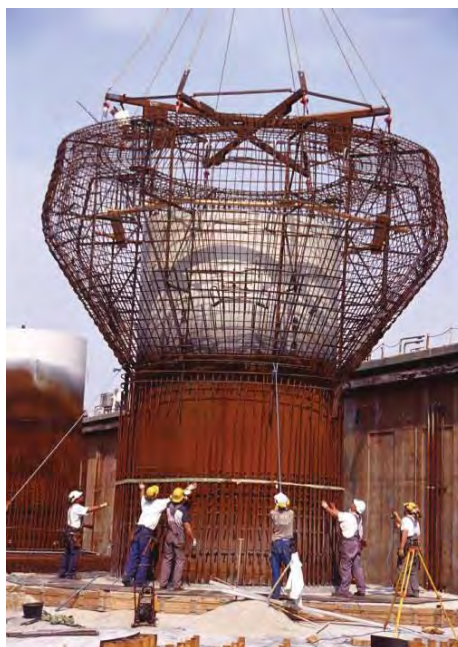
Figure 6-24: Middlegrunden Gravity Caisson construction in Dry Dock
