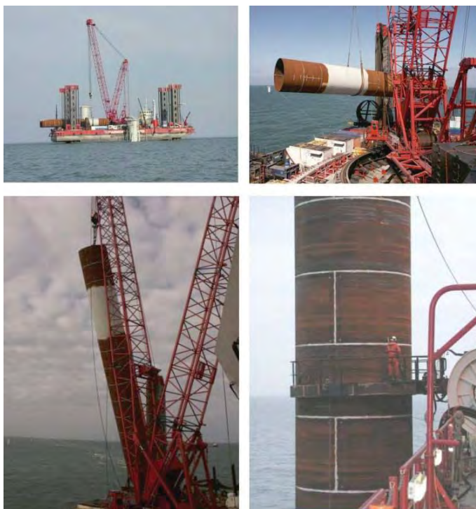
Figure 6-22: Monopile Installation at Arklow Bank, Ireland
