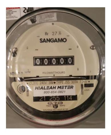
**N.1.e** Report the total meter reading number at the time the photograph was taken and specify the appropriate unit of generation (e.g., kWh): 0KWH
