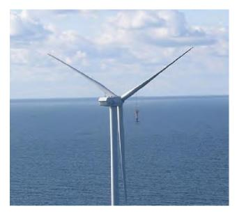
Fig. 15: Rotor in the "Y" position
