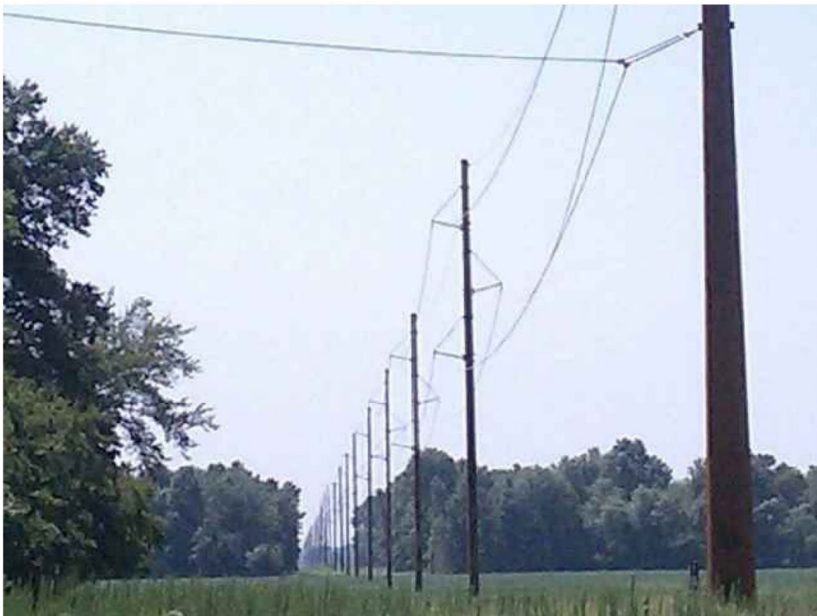
Diagram 04-1. Typical Tangent Structures
