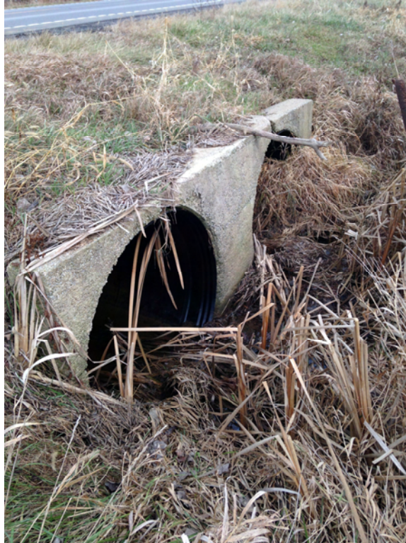
POI ID#543: Minor Cracking in headwalls
