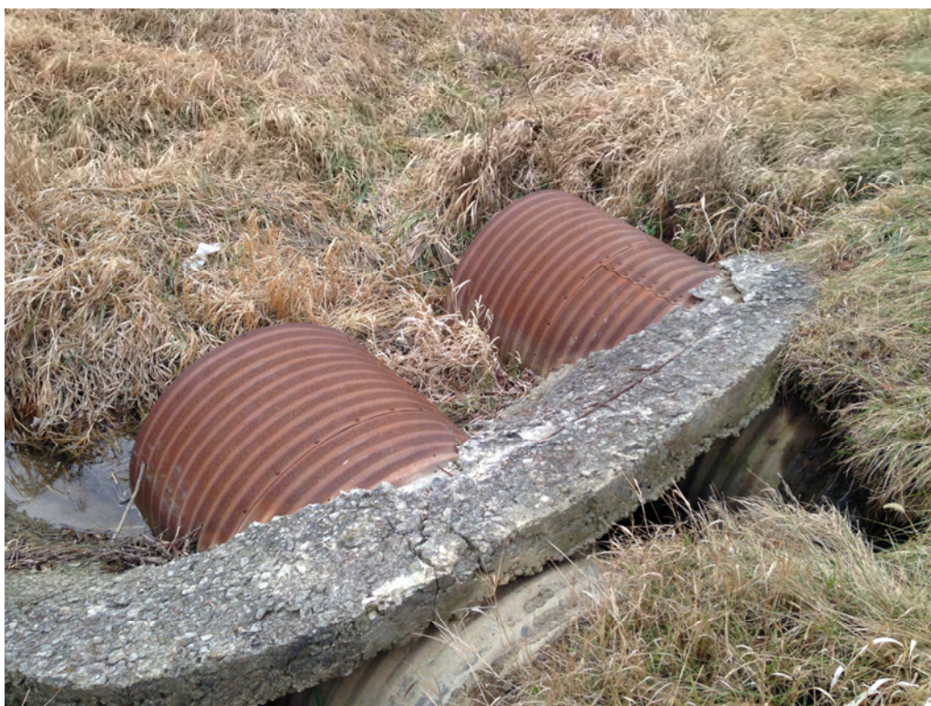
POI ID#531: Washout behind concrete collar
