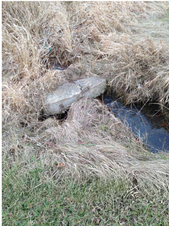
POI ID#601: Severe concrete cracking in collar
