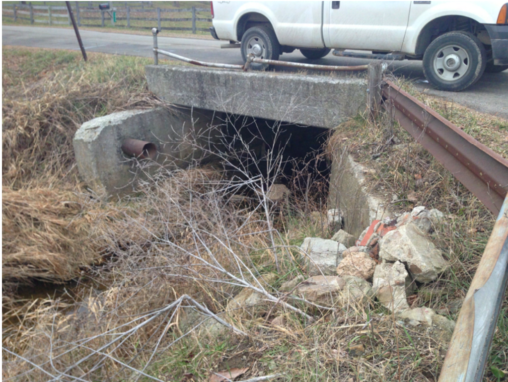
POI ID#378: Face of Box Culvert
