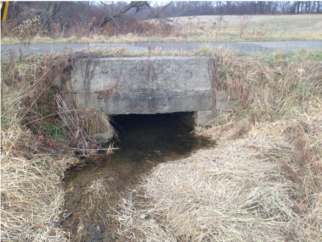
POI ID#374: Face of Box Culvert
