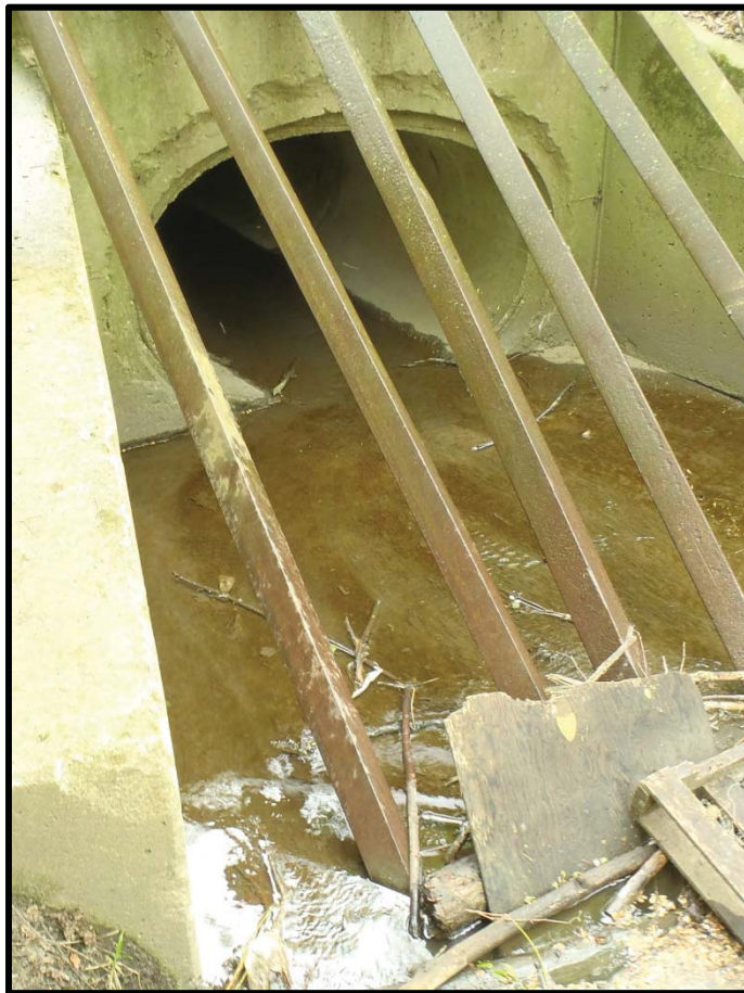
Photo 12. Stream 1 culvert inlet near Structure 16. This stream has been culverted and buried along the line until Structure 6. Image taken looking east on May 7, 2013.
