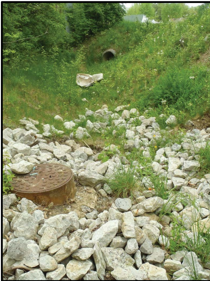
Photo 6. Drainage swale within the transmission line corridor with a culvert and drain near Structure 9. Image taken looking south on May 6, 2013.
