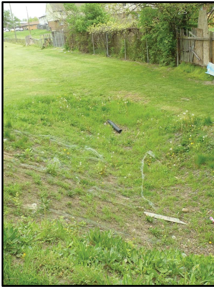
Photo 7. Drainage swale with discharge pipe within the transmission line corridor. Image taken looking north on May 6, 2013.
