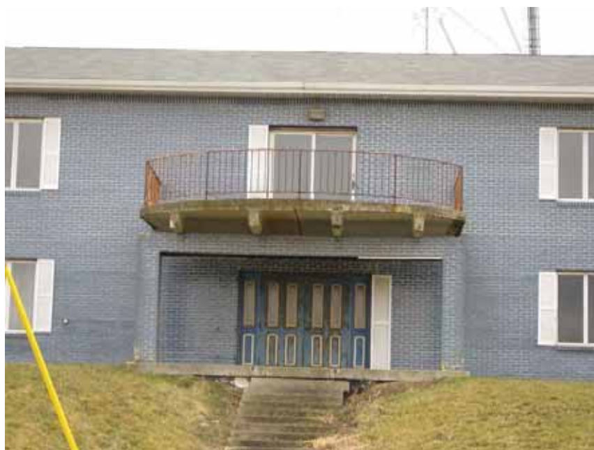
Photo 240. Cantilevered concrete T-beam/slab over porte-cochere
