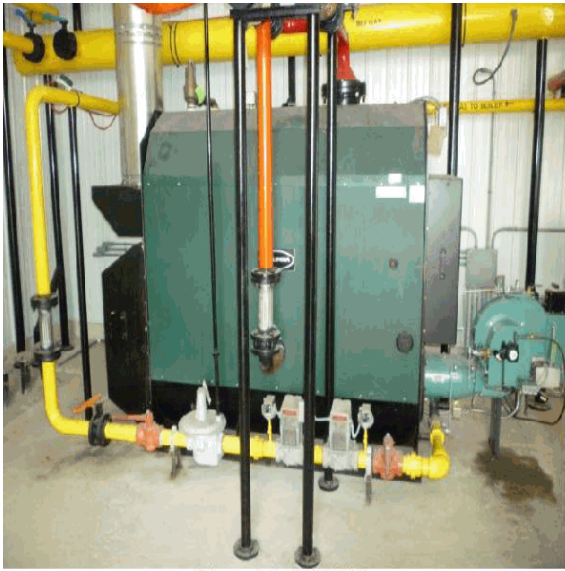
Digester boiler (8/23/2010)
