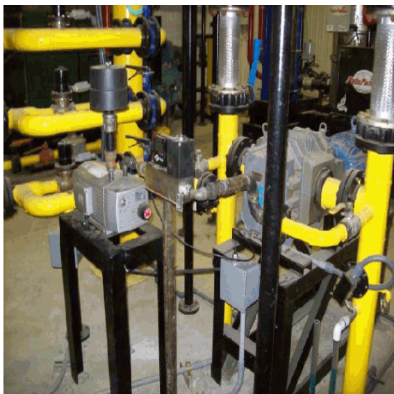
Digester H 2 S reduction system (9/23/2010)
