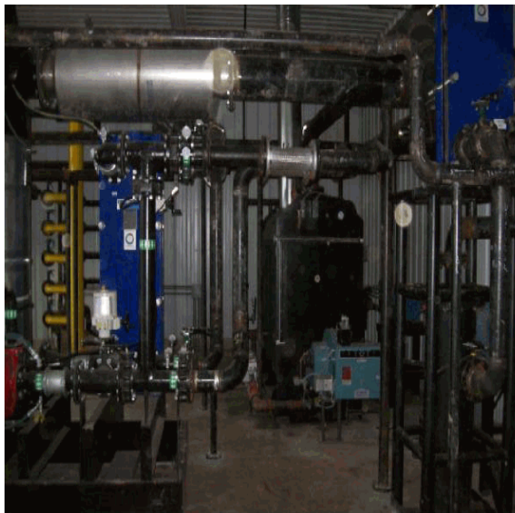
Digester boiler (5/13/2010)
