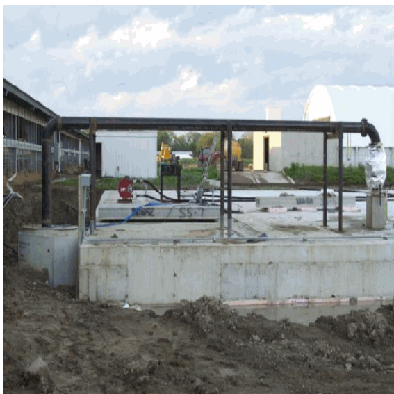
Digester gas piping (5/13/2010)
