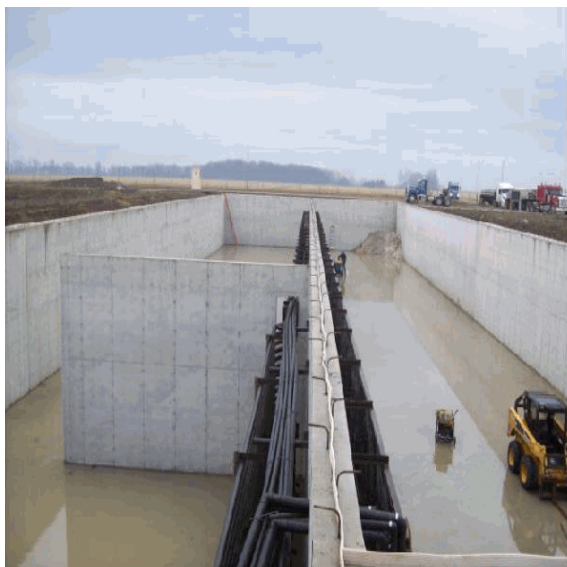
Digester heating racks (3/10/2010)
