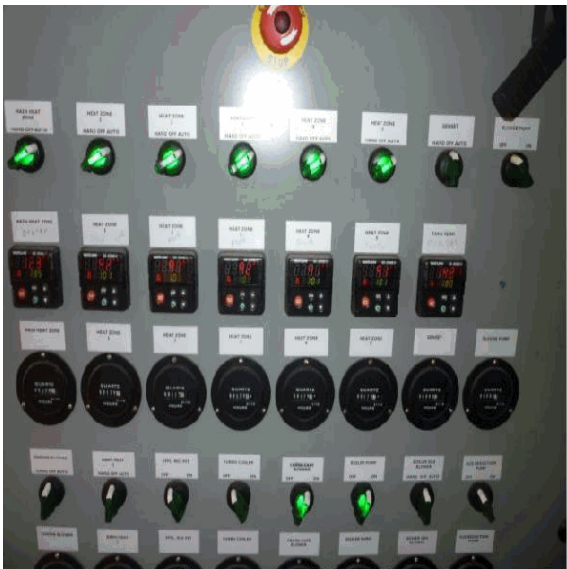
Digester control panel (8/23/2010)
