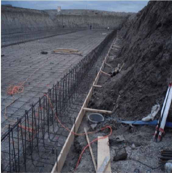
Digester floor rebar placement (11/11/2009)
