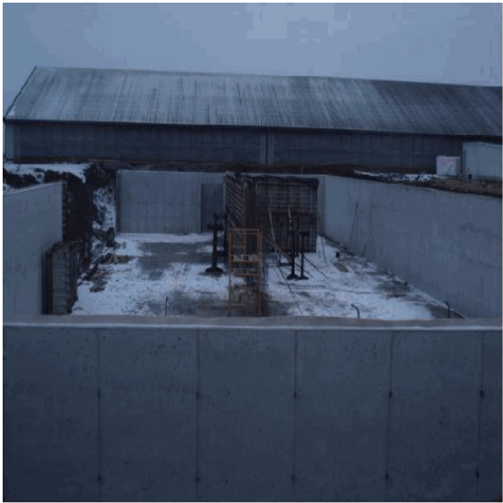
Digester wall construction (2/03/2010)
