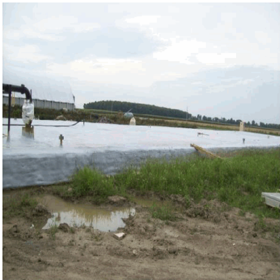
Digester cover insulation (7/16/2010)
