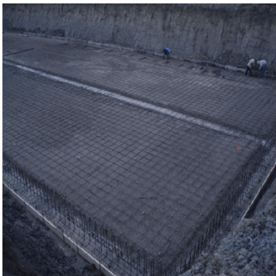
Digester floor rebar placement (11/04/2009)
