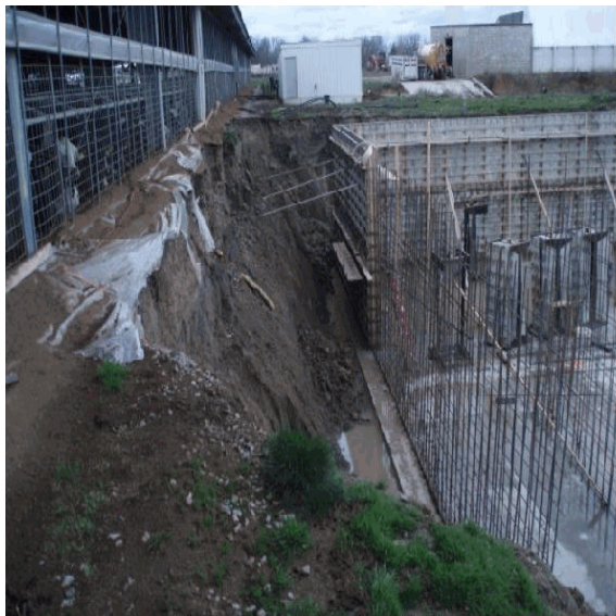
Digester wall construction (11/30/2009)
