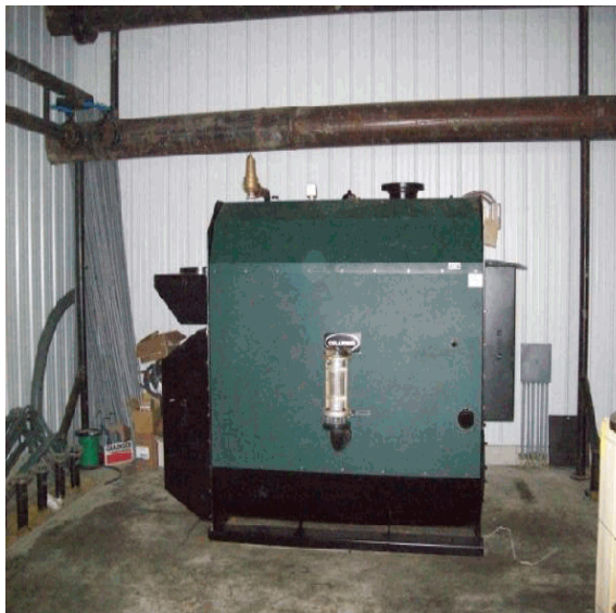
Digester boiler (3/10/2010)
