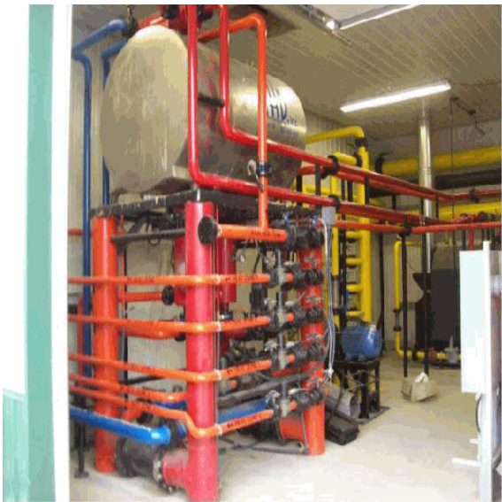
Digester heating system (7/16/2010)
