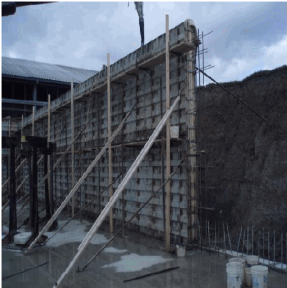
Digester wall construction (11/30/2009)
