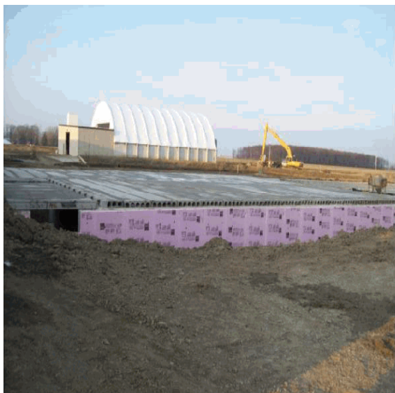
Digester cover installation (3/10/2010)
