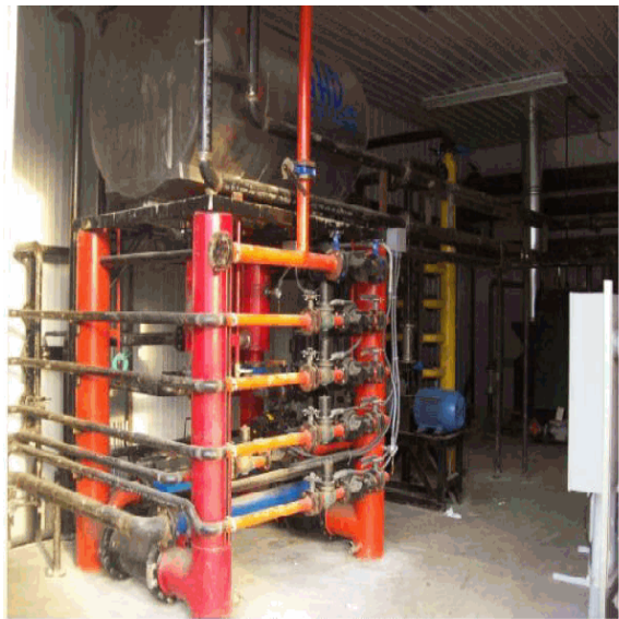
Digester heating system (5/13/2010)
