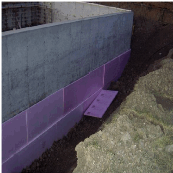
Digester wall insulation (12/04/2009)
