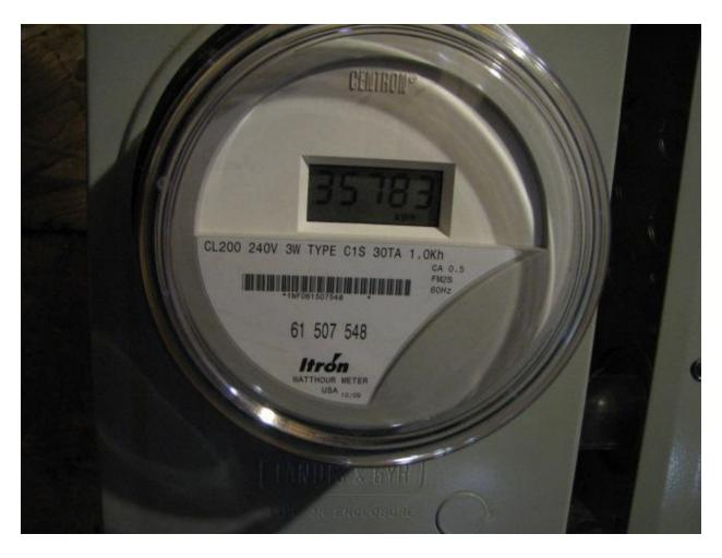
Report the total meter reading number at the time the photograph was taken and specify the appropriate unit of generation (e.g., kWh): 35,783
