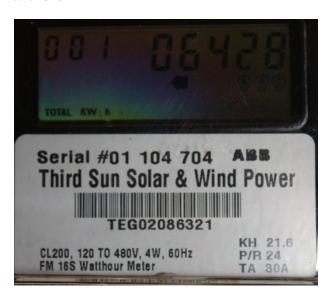
The total output of the inverters from 1/6/2010 - 7/2/2010 was 8,860 kWh. The total usage recorded by the meter from installation on 3/23/2010 - 7/2/2010 was 6,428 kWh. We will calculate the SRECs generated from 1/6/2010 - 3/23/2010 by subtracting the meter reading from the inverter reading for a total of 2,432 (8,860 – 6,428 = 2,432 kWh). This 2,432 kWh will be recorded in addition to the calculations from reply #1.
