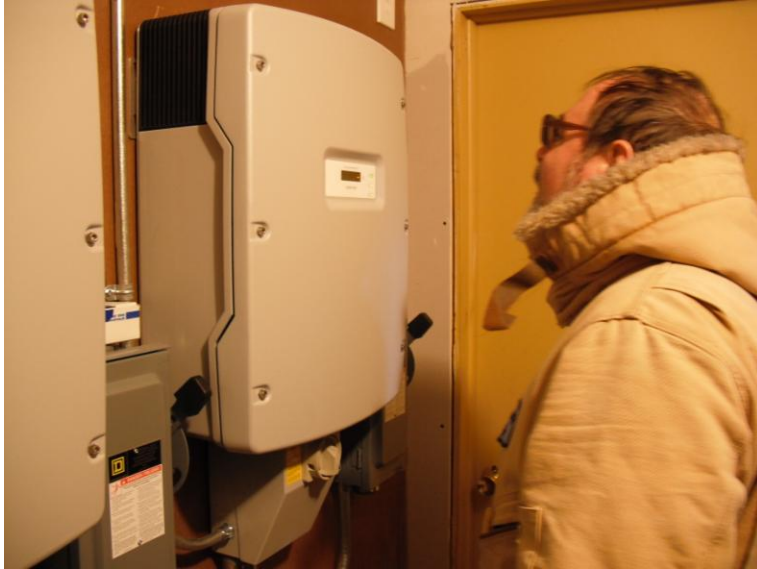
Viewing one of the Sunny Boy Inverters
