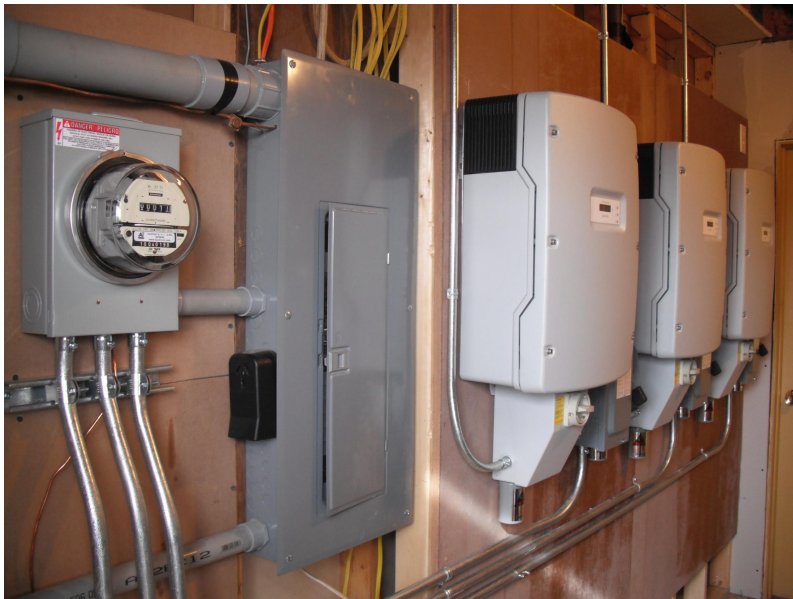
Utility room showing the 3 inverters, main AC panel and the Power Meter for just the solar array. The three inputs are from the 3 inverters.
