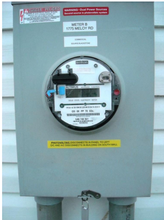
SOLARIS BLACKSTONE 10.5 KW ARRAY Commercial Meter / Siemens Bi-Directional Meter Taken 8-26-2009
