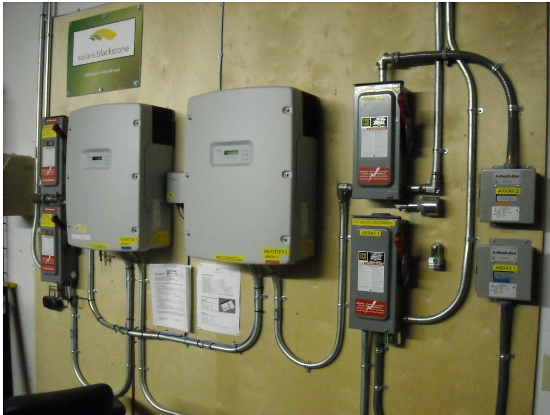
SOLARIS BLACKSTONE 10.5 KW ARRAY Switchgear, Inverters, Meters, Web-box Taken 8-26-2009
