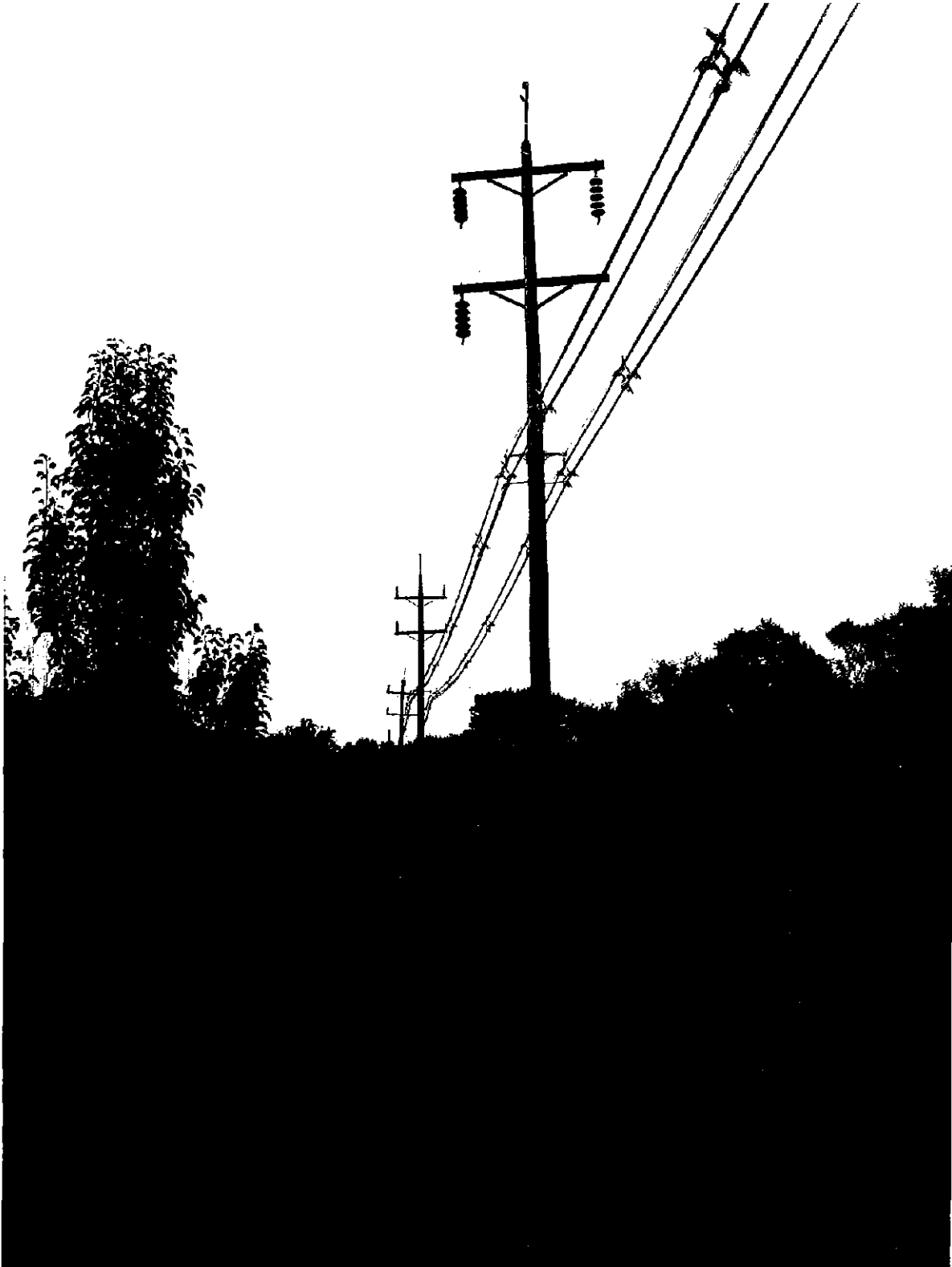
Figure 5. Transmission line that extends from east to west across the subject site. Substation 13's position will be to the left of the bottom of this photograph.
