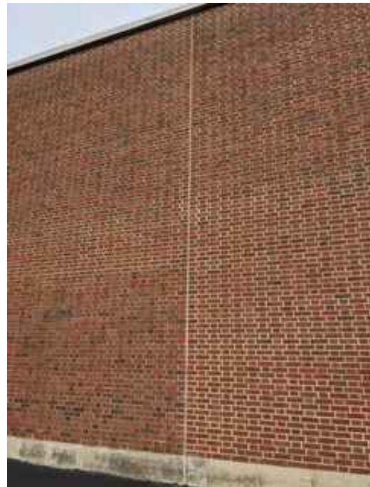
Control Joint Between Additions
