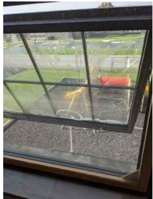
Window with Peeling Coating
