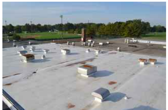
TPO with Signs of Past Ponding
