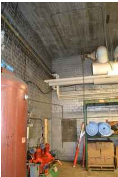
Precast Concrete Plank Deck
