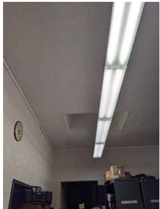
Screw Spline Ceiling Tile
