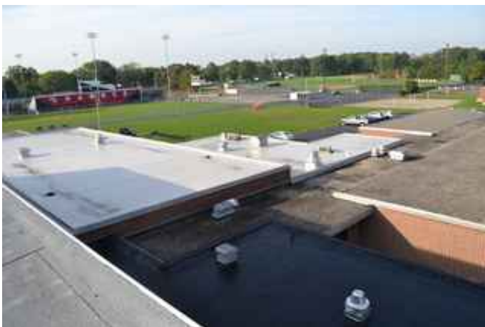
EPDM, TPO, and Ballasted Roofing
