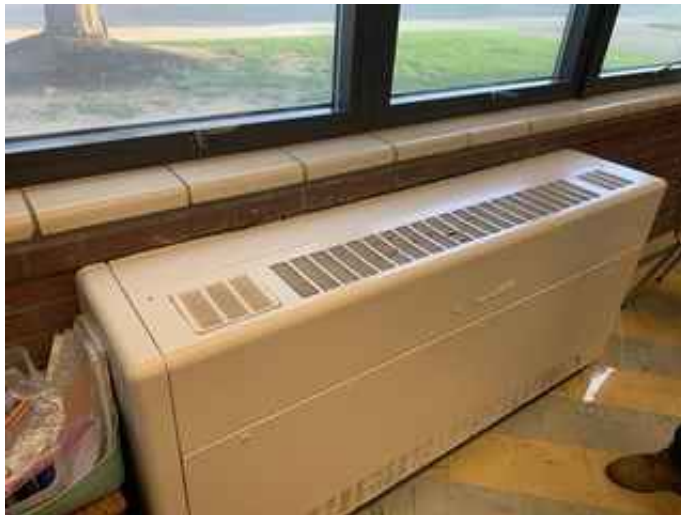
steam unit ventilator
