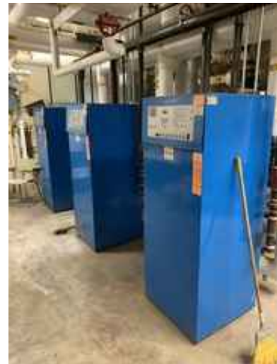
Hot water boiler (west building)
