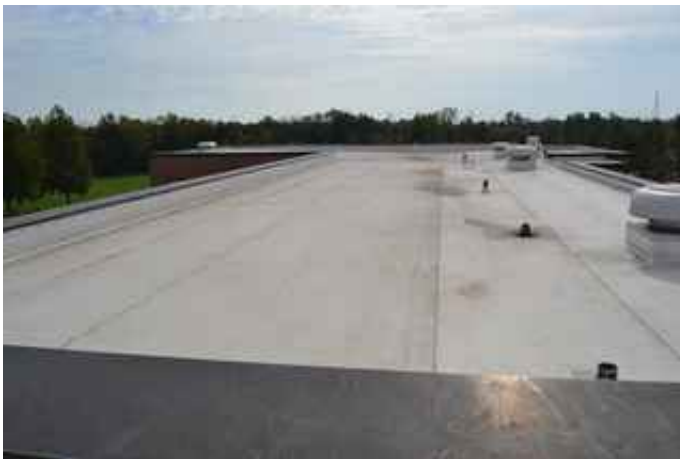
TPO Roofing with Evidence of Previous Ponding
