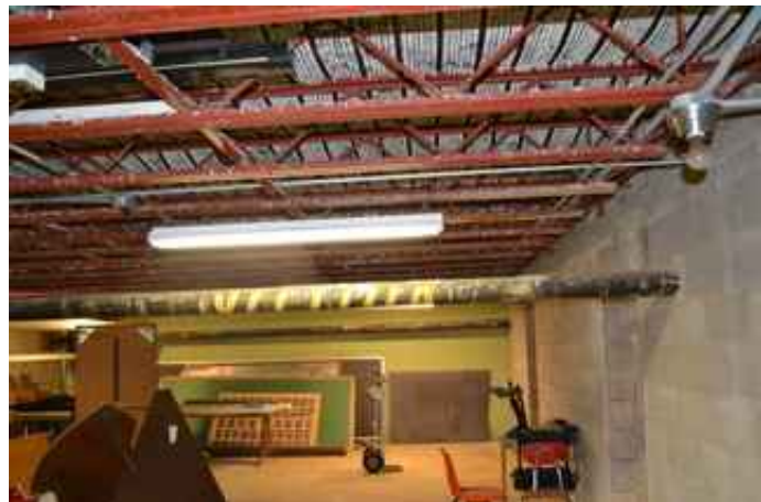
Precast Gypsum Deck on Steel Joists
