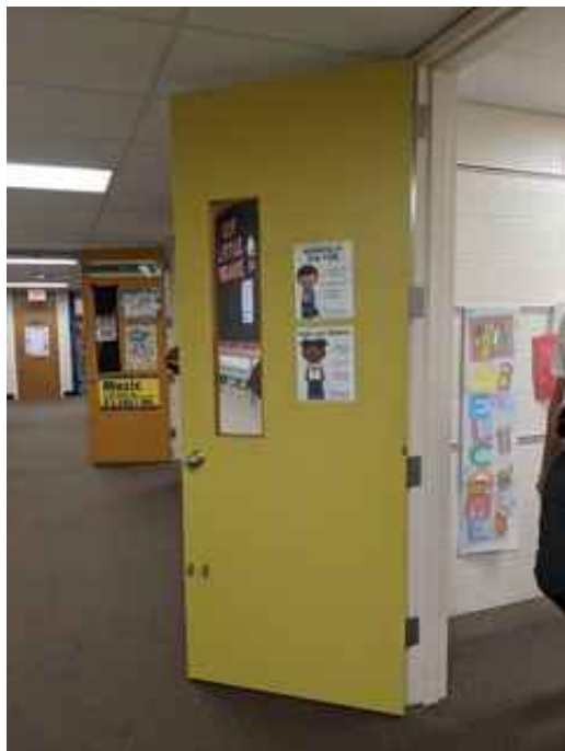
Interior Door Without ADA Compliant Hardware
