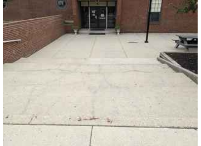
Concrete Steps Needing Repair
