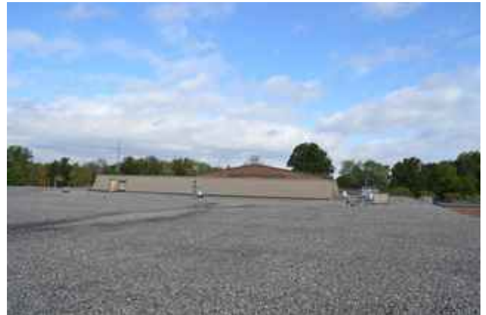
Ballasted Roofing
