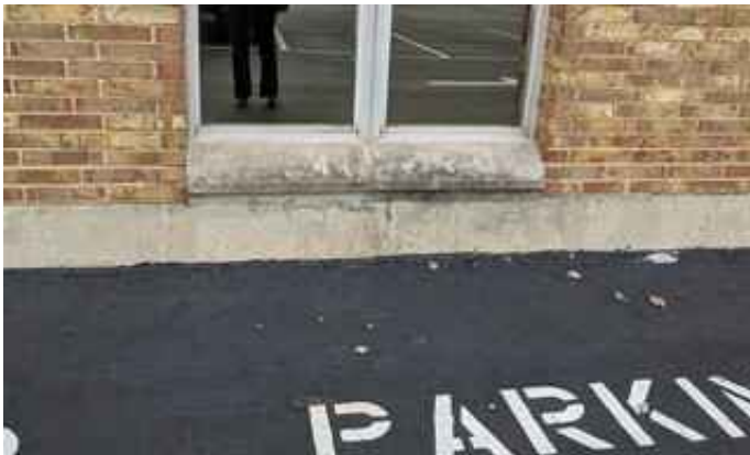
Window Sills to be Replaced
