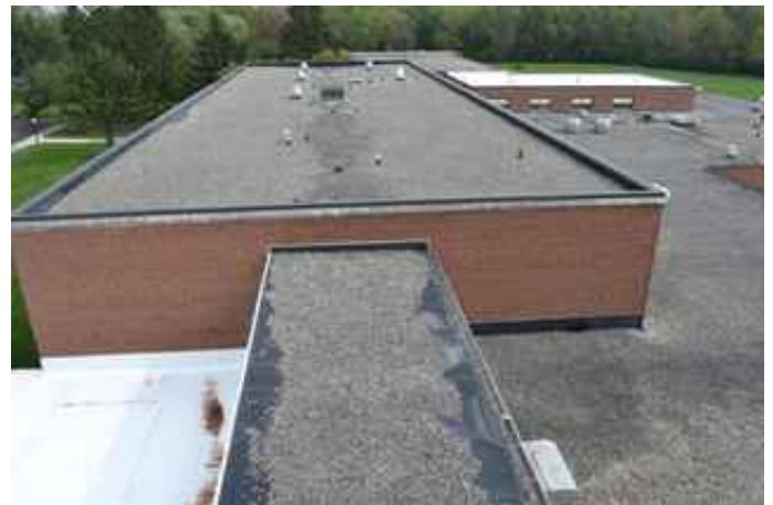
Ballasted Roofing
