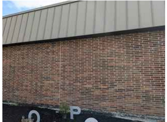
Exterior Masonry and Control Joint
