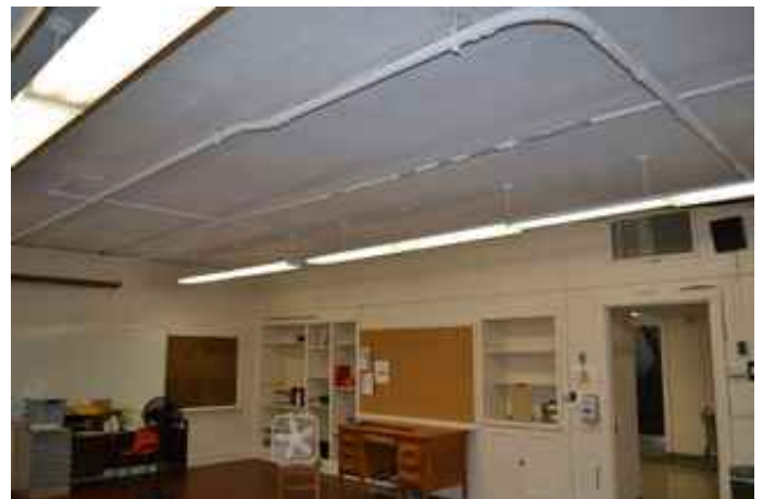
Screw Spline Ceiling Tile
