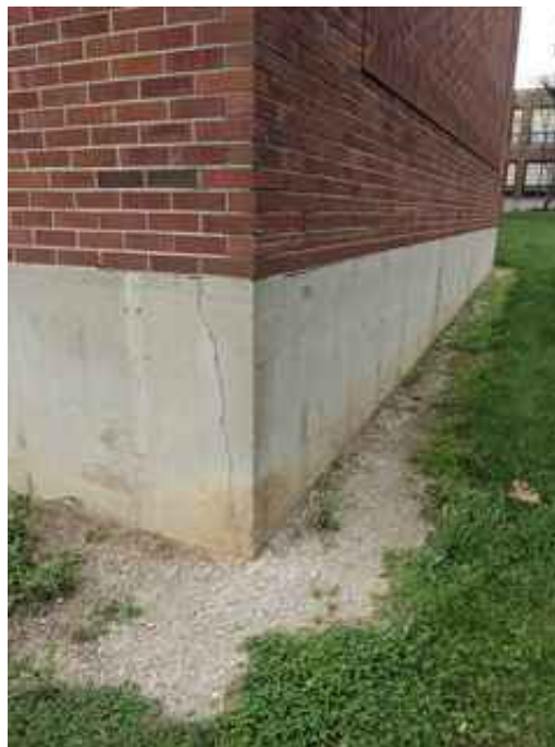
Foundation Crack
