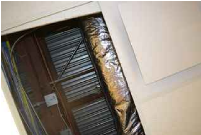
Metal Deck and Steel Joists
