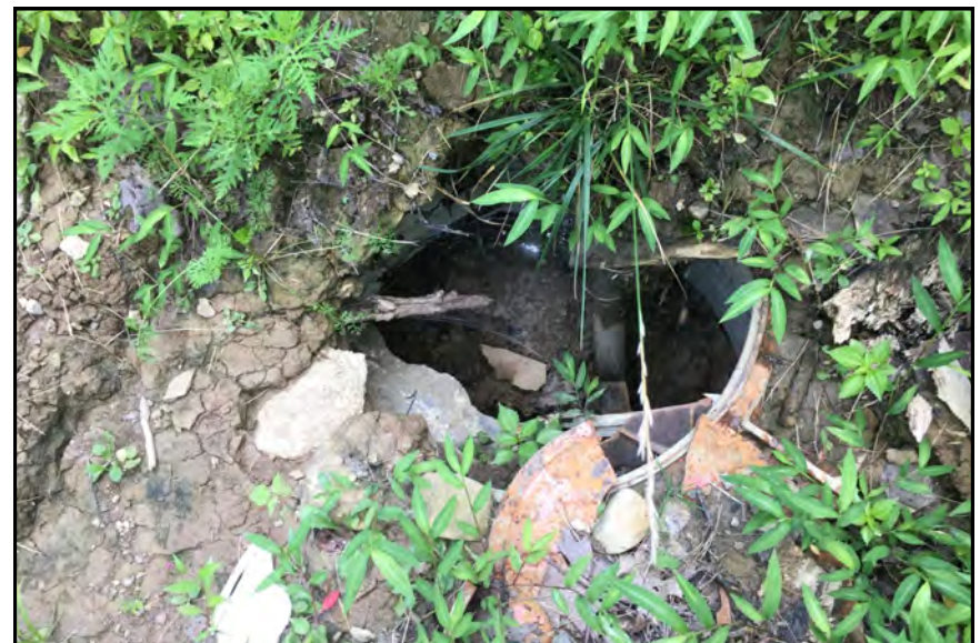
Photo 8: Manhole, located in Ditch 1.
