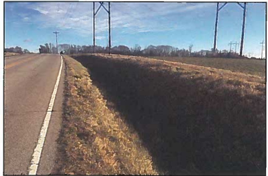
Photo 22: Roadside ditch along Hamilton Road, looking Northeast.
