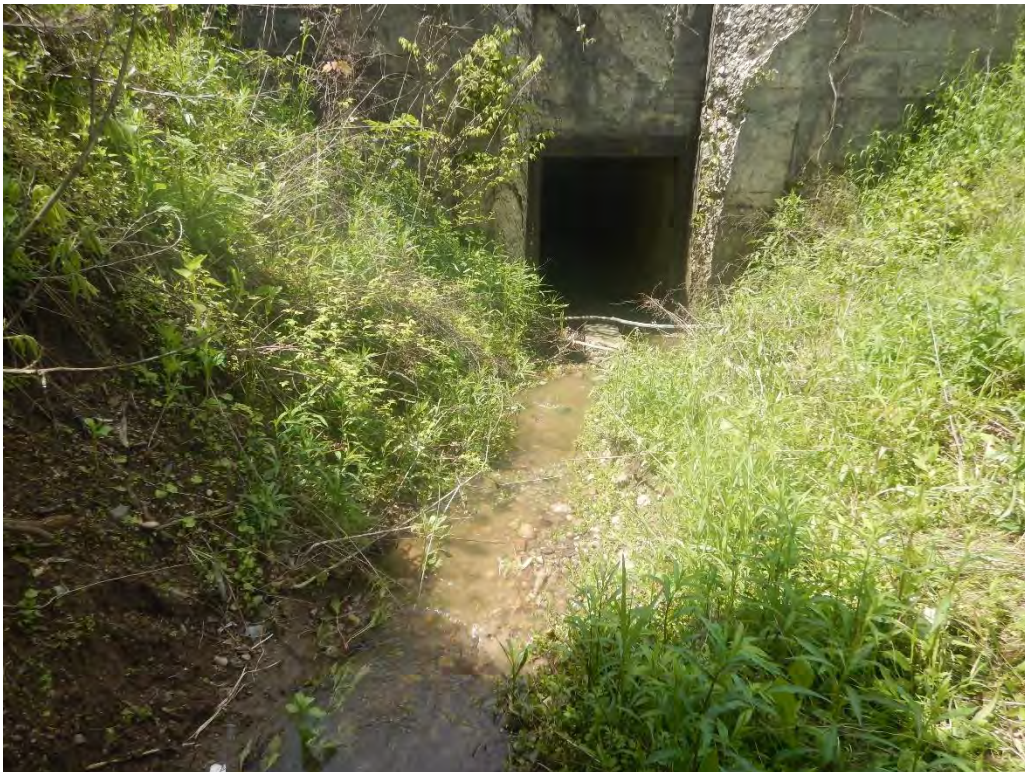
Photograph 8: View downstream of KLF_Stream08 (INT)
