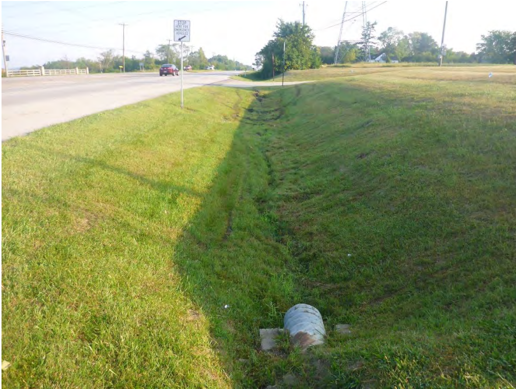
Photograph 13: View North of KLF_Wetland01 (PEM)
