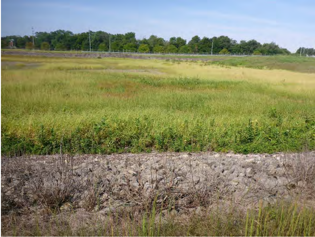
Photograph 5 – KLF_BH05 view West (BC-4)
