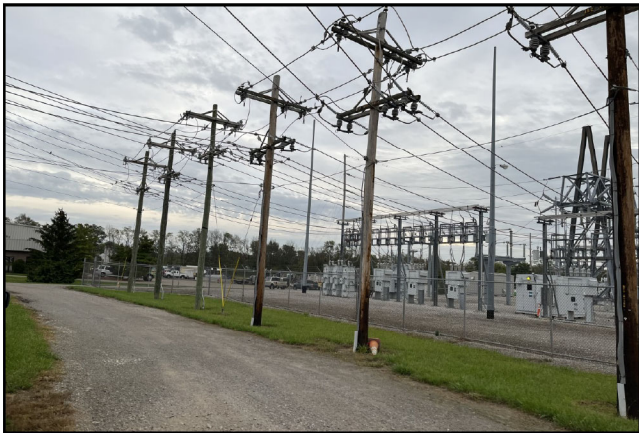
Photo 1: Project Area overview; existing substation and transmission lines.
