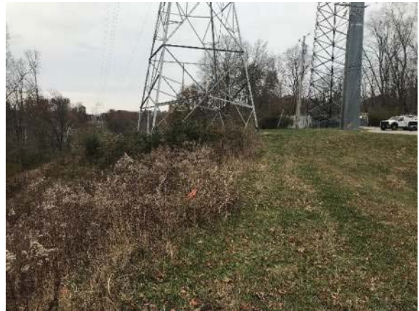
Photograph 4. Location of Str. HL905. Looking north. (November 14, 2018)
