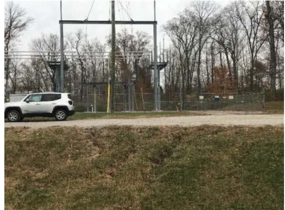
Photograph 8: Looking east towards Str. HL904 with substation beyond. (November 14, 2018)
