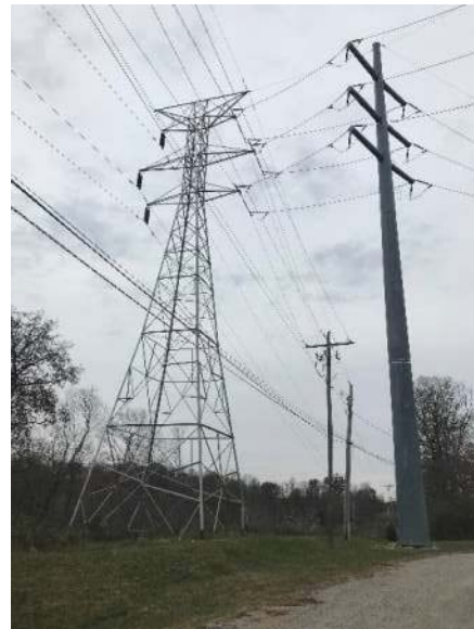
Photograph 16: Existing tower structure near proposed structures (HL900 – HL905). (November 14, 2018)
