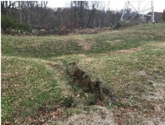
Photograph 3. Severe stormwater erosion, adjacent to gravel access road. (November 14, 2018)
