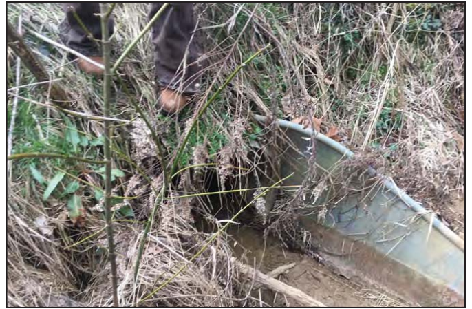
Photo 2. View of Stream 1 as it enters a culvert.
